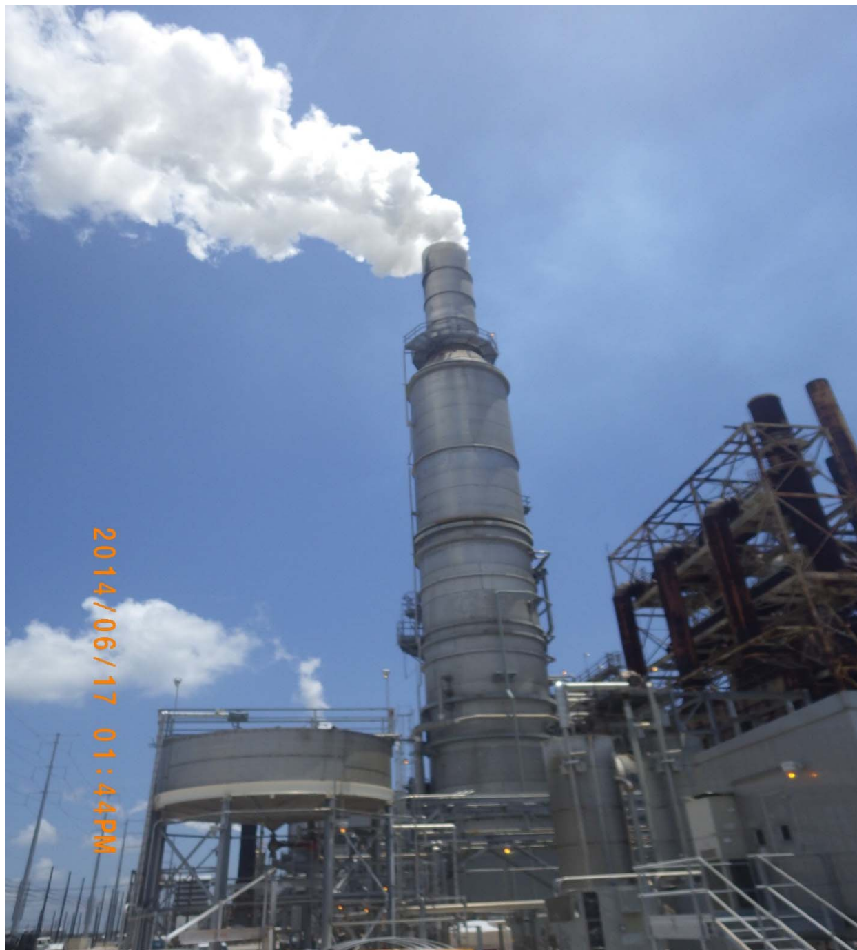
Fluidized Catalytic Cracking Unit (FCCU) 1241 Wet Gas Scrubber (WGS)
