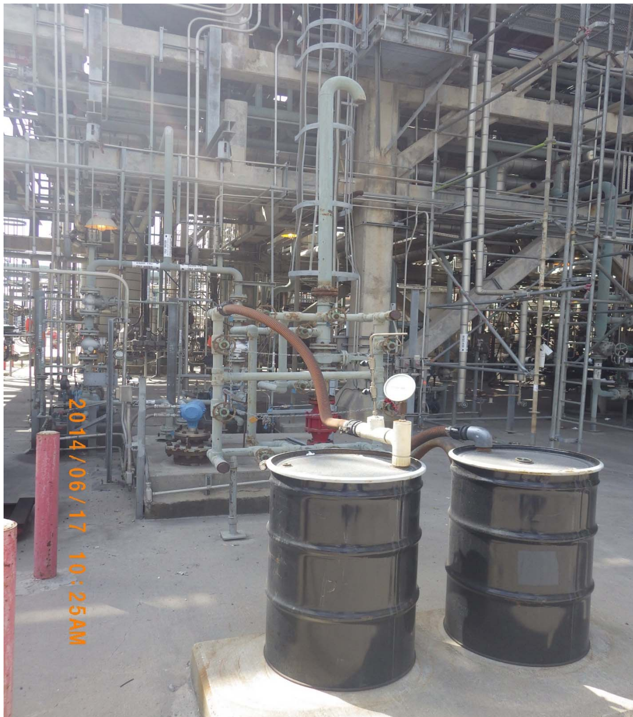
BWON Carbon Canisters arranged in series.
