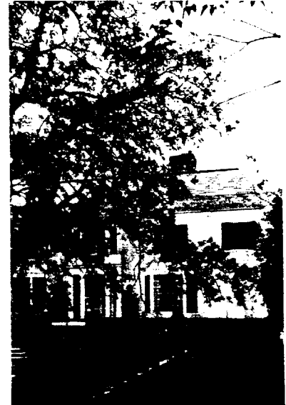
General view of the Purchase, N. Y., residence where sheet lead was used extensively for flashing and ornamental work
