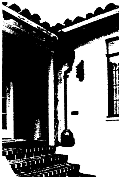
View of the front entry with lead gutters, leader and leaderhead, and ornamental lead lanterns
