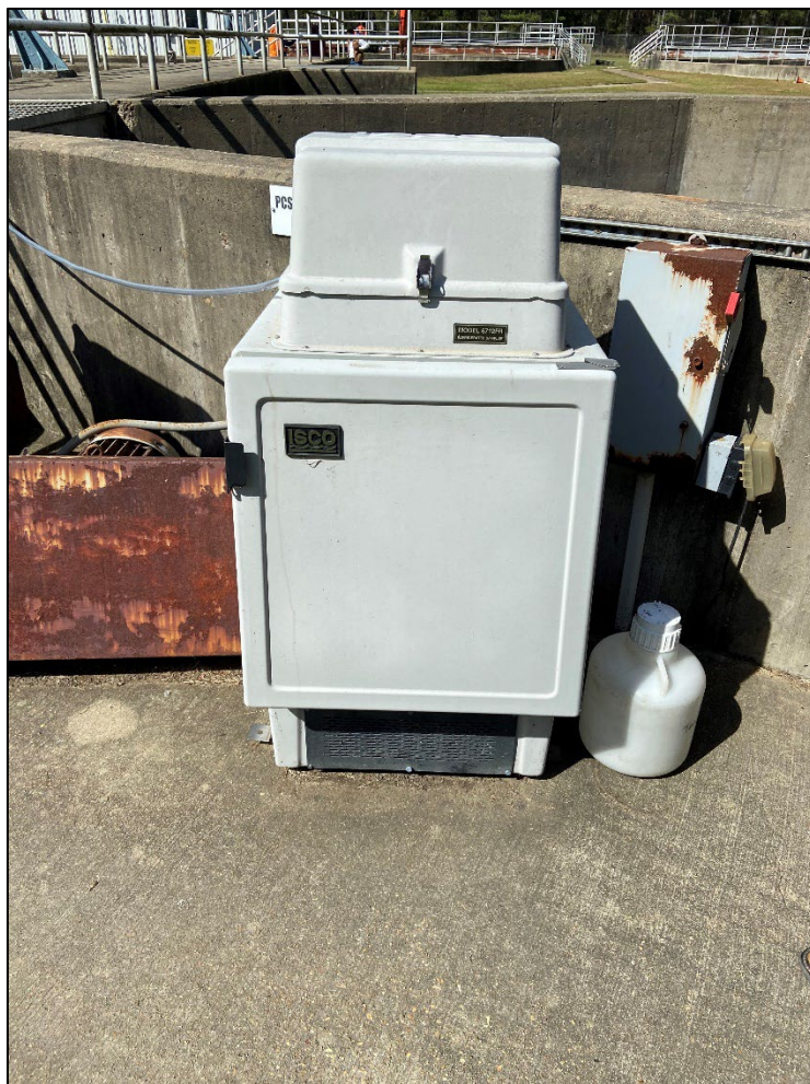
Photo 14: Effluent automatic sampler.
