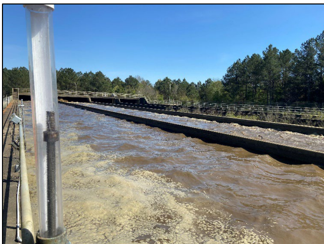
Photo 5: Oxidation ditch #1.
