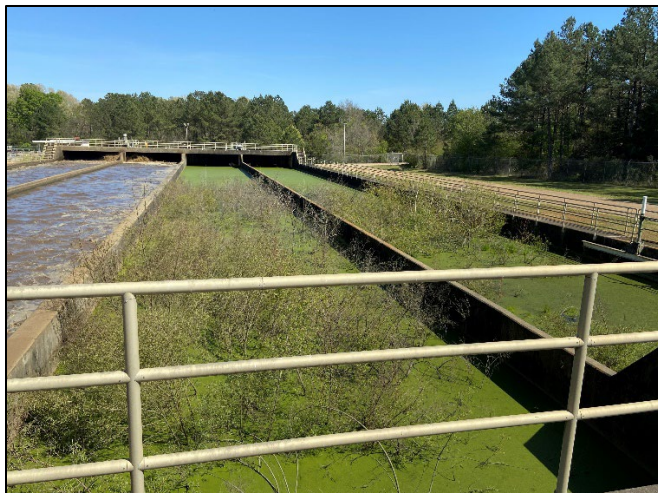
Photo 6: Oxidation ditch #2.
