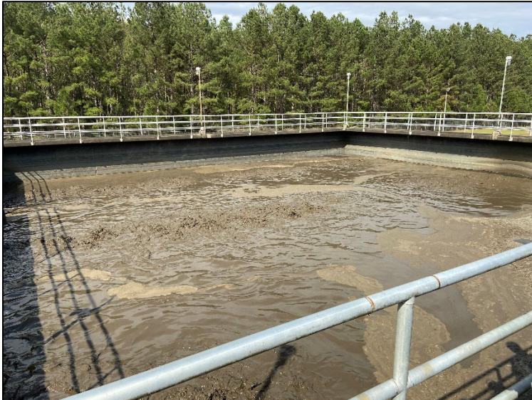
Photo 17: Sludge digester.
