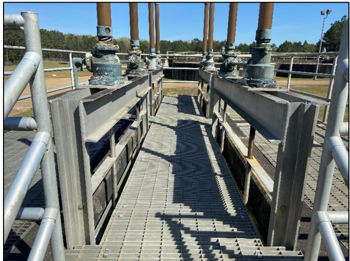
Photo 4: Splitter box to oxidation ditches.
