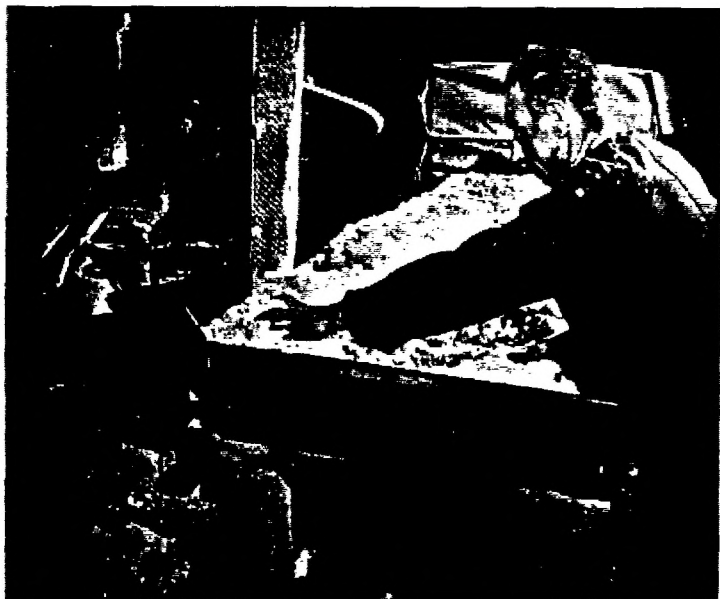
REFINING FIBER at loading bin of impact machine is Gerald Hahn. Various fibers are used, depending on the type of asbestos packing desired.
