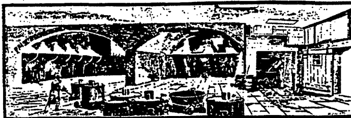
Melting rooms in the Newark factory of the Murphy Varnish Co.
