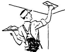
ACOUSTICAL PLASTER FINISH
