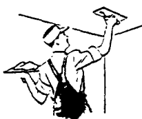
ACOUSTICAL PLASTER FINISH
