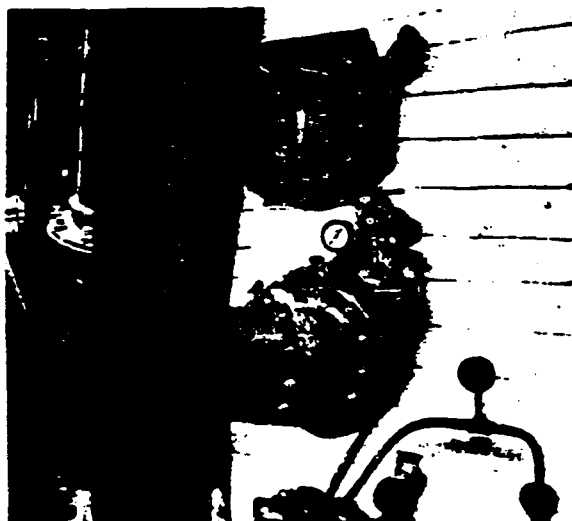
Refractory tile of boiler wall in place behind boiler tubes being backed up with R & I #14 Insulating Block.
