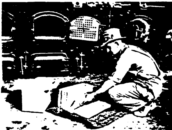
Six ready cut slices of R & I Plastic Fire Brick each 2" thick, removed from carton, easy to handle and apply.
