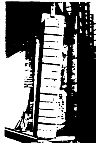
Coke oven door lined with blocks made of R & I Moldit Pier Cement. Moldit block doors of this type last three to four years—and even longer.
