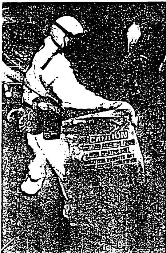
Asbestos removal may pick up in private buildings.
