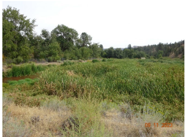
Photograph #08 (DSC03532) Description: North solids drying bed. The drying bed had standing water as well as a gravel bottom and vegetation growth throughout.
