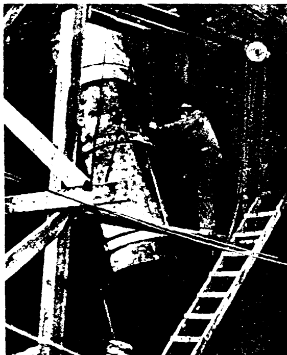
Below, preparing to remove the mandrel from a completed section of the lead duct. Note that steel straps which provide both stiffening and support are secured to the duct and sealed off from corrosive atmosphere by sheet lead covering burned to the duct wall.
