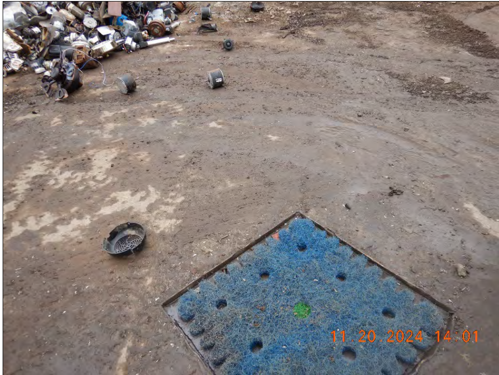
Photograph 3. DSCN0715.JPG View of the storm drain inlet shown in Photograph 2. A filter pad was installed at the storm drain inlet.
