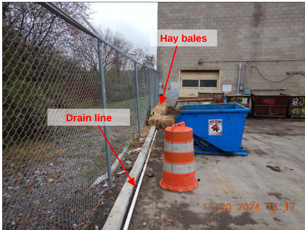
Photograph 13. DSCN0725.JPG View of the drain line for the oil/water separator. The line ends at hay bales between the oil/water separator and the non-ferrous peddlers building.
