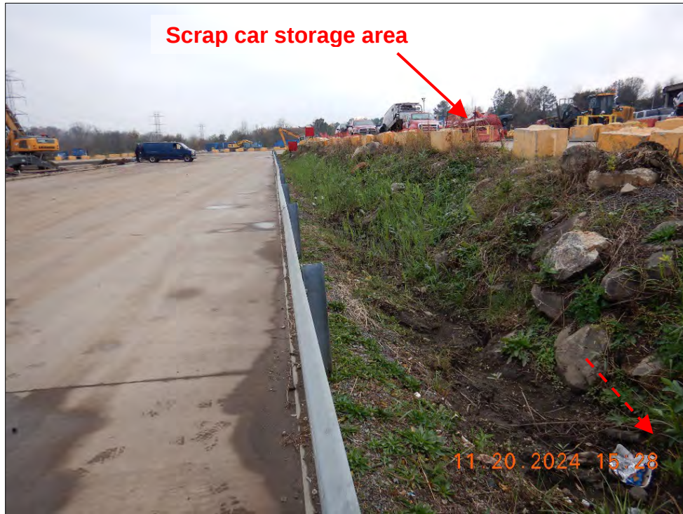
Photograph 47. DSCN0767.JPG View, facing south, of the ditch that conveys stormwater to the storm drain shown in Photographs 43–45. The SWPPP site map does not identify stormwater drainage flow inside this ditch. The SWPPP site map documents stormwater runoff flowing across this ditch from west to east.
