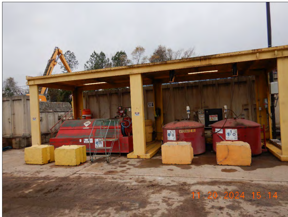
Photograph 40. DSCN0759.JPG View of diesel fuel, hydraulic oil, and engine oil ASTs at the maintenance shop.
