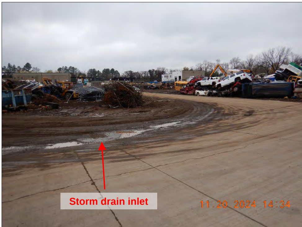
Photograph 20. DSCN0734.JPG View of a storm drain inlet on the east side of the scrap storage/sorting area. A BMP was not installed at the inlet.
