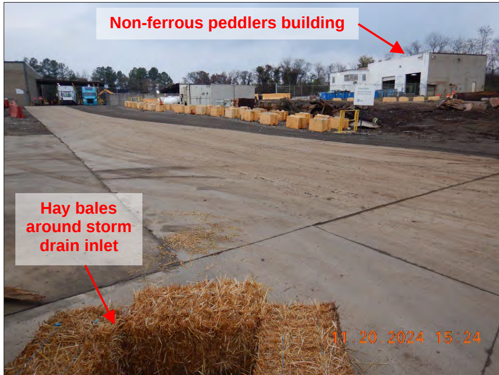
Photograph 43. DSCN0763.JPG View of a storm drain in the scrap storage/sorting area that was not identified on the SWPPP site map.
