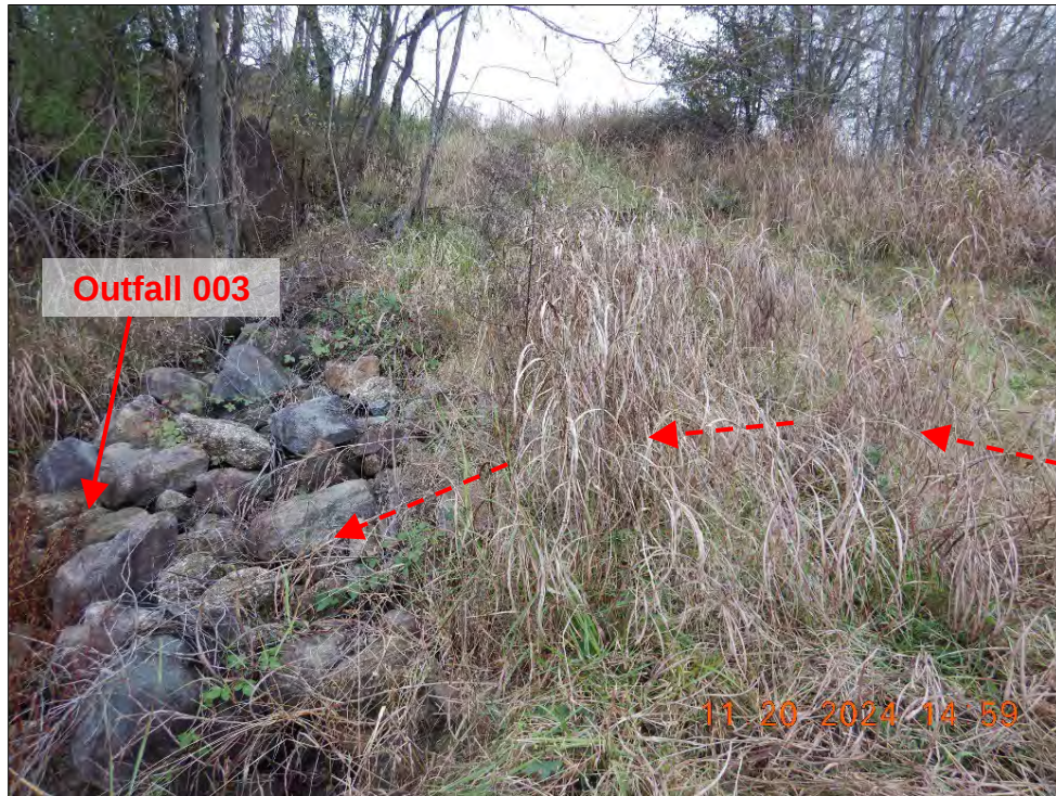
Photograph 35. DSCN0752.JPG View, facing west, of Outfall 003. Stormwater flows from the north to Outfall 003. The area directly north of the outfall is raised above the ditch that flows to the outfall. The Facility was not discharging from Outfall 003 at the time of the inspection.
