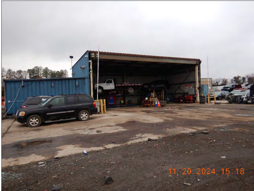
Photograph 41. DSCN0760.JPG View of the SEDA system used for vehicle de-pollution prior to crushing.
