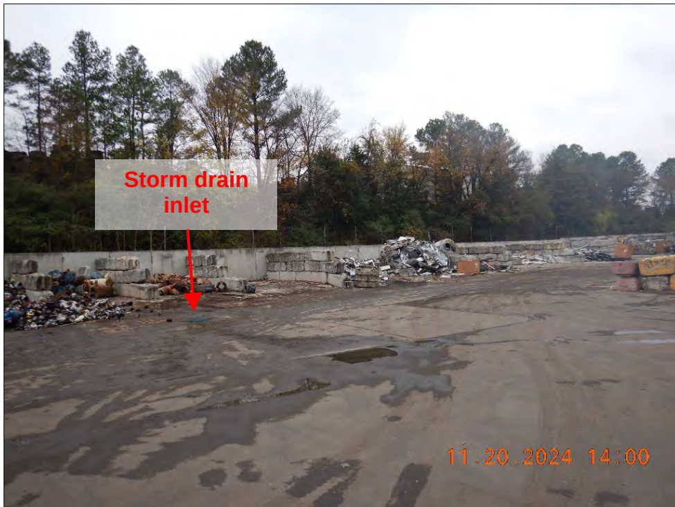
Photograph 2. DSCN0714.JPG Additional view of the scrap storage area in the northwest portion of the Facility.
