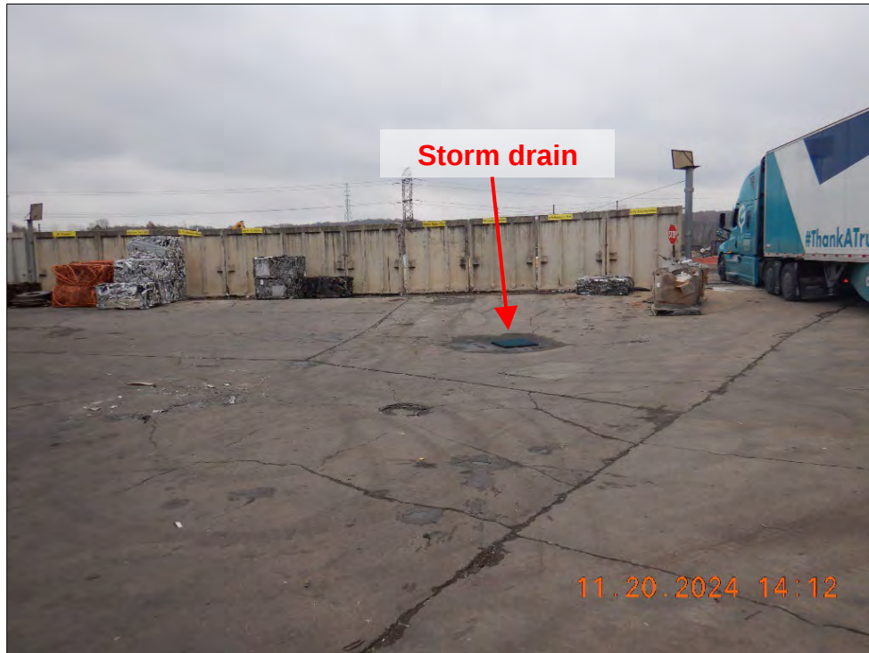
Photograph 7. DSCN0719.JPG View of a storm drain inlet southeast of the baler.
