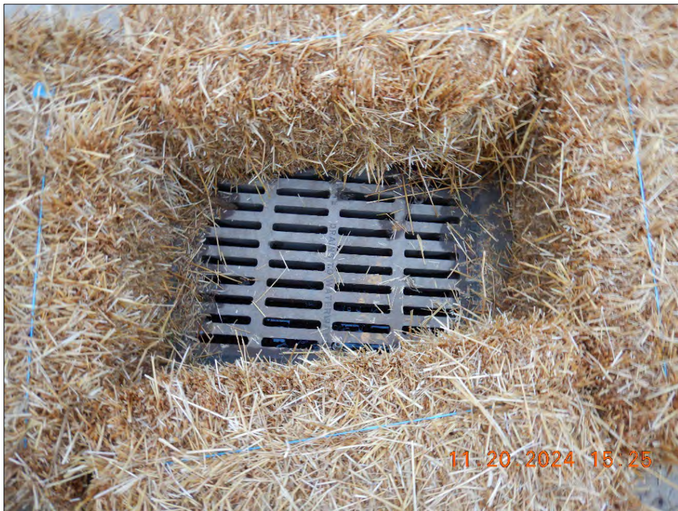
Photograph 44. DSCN0764.JPG Close-up view of the storm drain inlet shown in Photograph 43.
