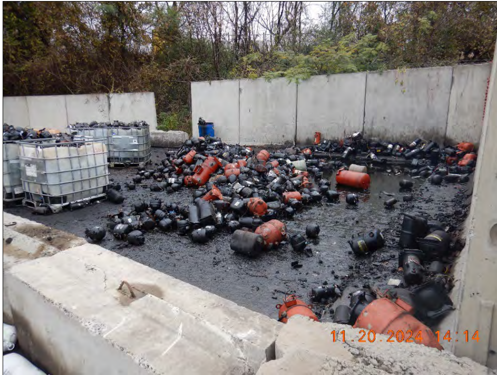
Photograph 9. DSCN0721.JPG View of the sealed components area. The area was not covered. The area slopes toward a sump that is pumped to an oil/water separator.
