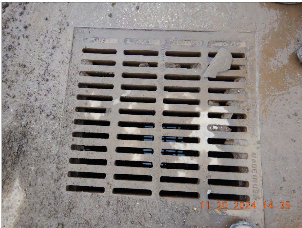
Photograph 22. DSCN0736.JPG Close-up view of the storm drain inlet shown in Photographs 20 and 21. Note sediment adjacent to and inside the grating of the storm drain inlet.
