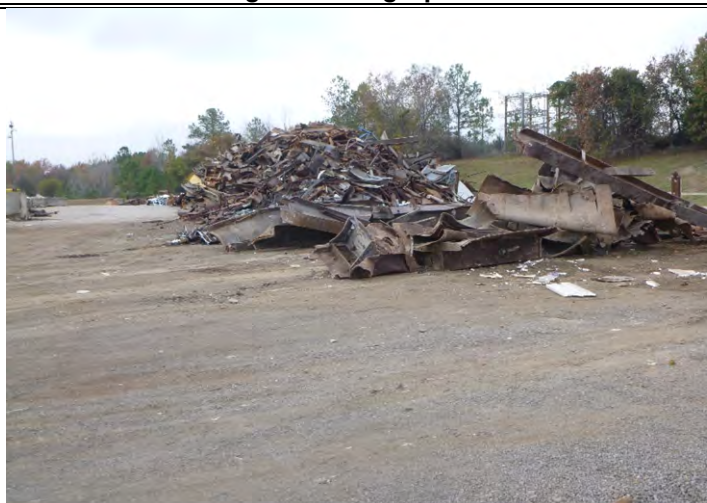
Photograph 2: Metal stockpile to be removed from site via rail.
