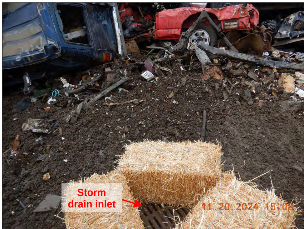
Photograph 30. DSCN0757.JPG View of the storm drain inlet, shown in Photograph 29, that was uncovered by Facility staff during the inspection.
