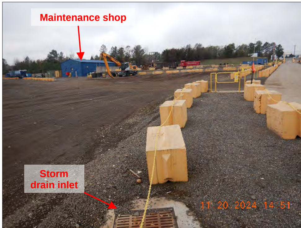
Photograph 37. DSCN0748.JPG View of a storm drain inlet south of the scrap storage/sorting area, on the south side of the road that runs along the south and east side of the scrap storage/sorting area. This storm drain inlet was not identified on the SWPPP site map.
