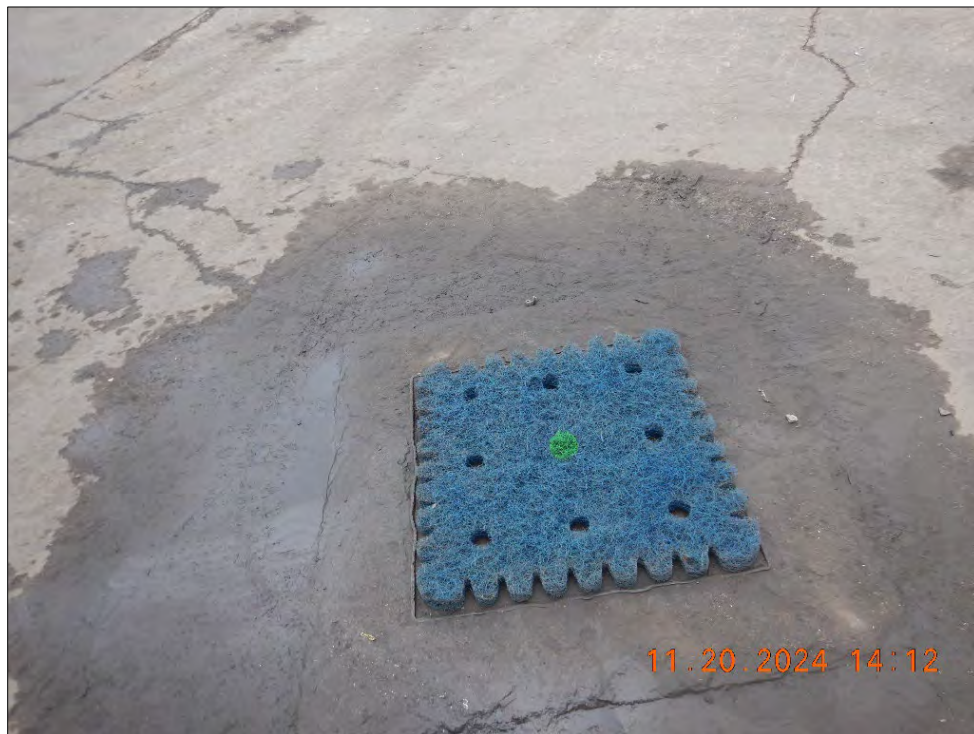
Photograph 8. DSCN0720.JPG View of the storm drain inlet shown in Photograph 7. A filter pad was installed on the storm drain inlet.
