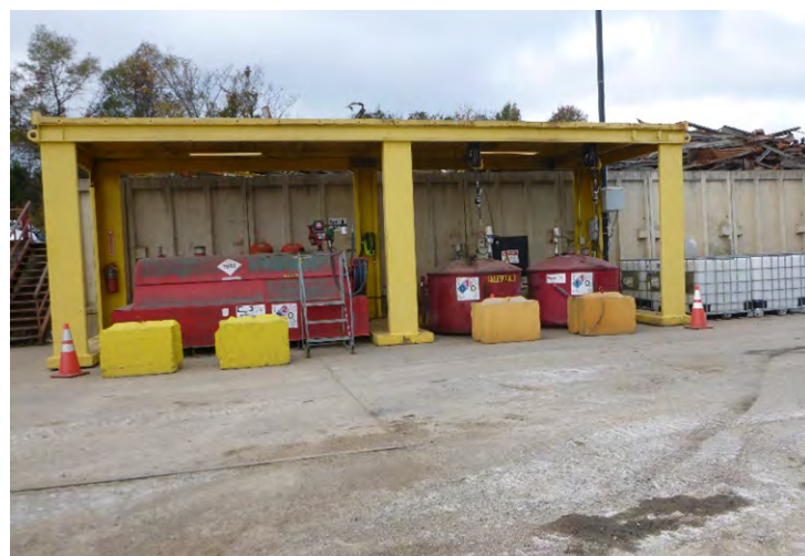
Photograph 3: Oil tanks located near the maintenance building.
