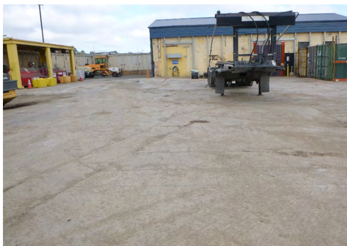
Photograph 4: Concrete pad used for equipment maintenance.
