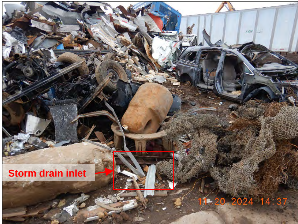
Photograph 23. DSCN0737.JPG View of a storm drain inlet on the east side of the scrap storage/sorting area. The inlet was covered with scrap material and lacked a BMP. Facility staff removed the scrap material and placed hay bales around this inlet during the inspection.
