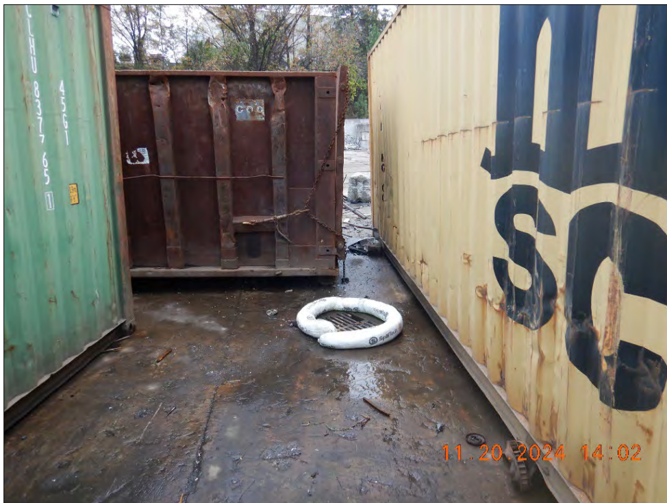
Photograph 4. DSCN0716.JPG View of a storm drain inlet in the scrap storage area. A filter sock was installed at the storm drain inlet.
