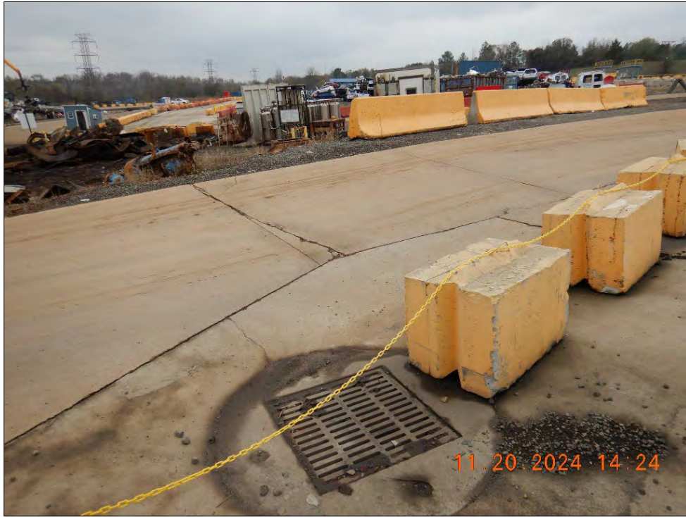
Photograph 15. DSCN0726.JPG View, facing south, of the storm drain inlet shown in Photograph 14.
