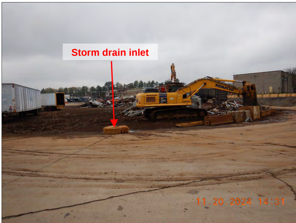
Photograph 18. DSCN0732.JPG View of a storm drain inlet on the east side of the scrap storage/sorting area. Hay bales were installed around the storm drain inlet.
