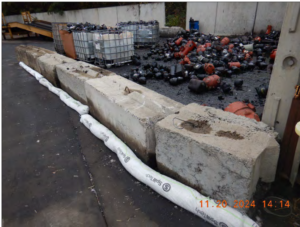
Photograph 10. DSCN0722.JPG Additional view of the sealed components area. Absorbent socks were installed along the concrete containment barrier on the south side of the area. Staining was observed on the concrete barrier and the impervious ground surface outside of the containment structures.
