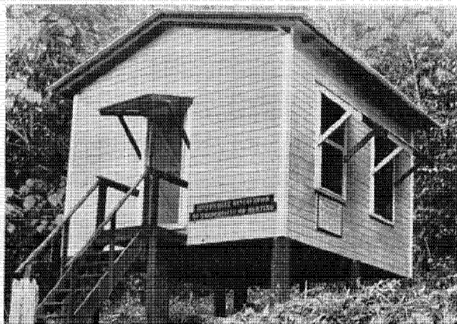
● The Termite Test House at Barro Colorado Island, Panama Canal Zone, stands on creosoted timbers, but the building itself was built of wood pressure treated with zinc chloride. After nine years' exposure it is still in a perfect state of preservation.
