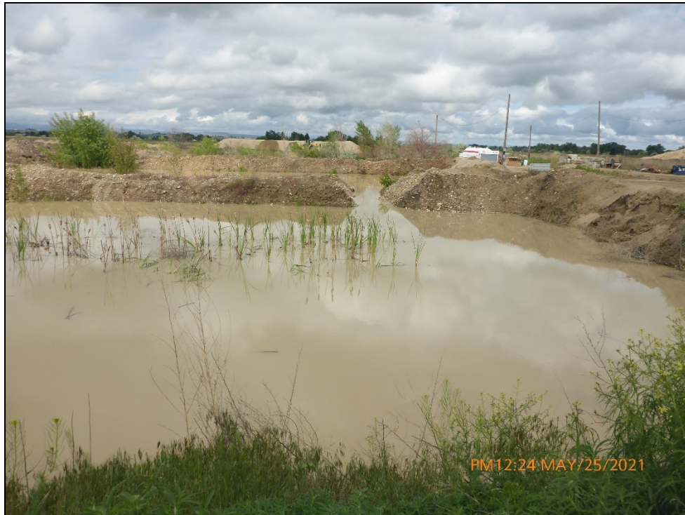
Photograph 19. View of the third and fourth wash water settling ponds.
