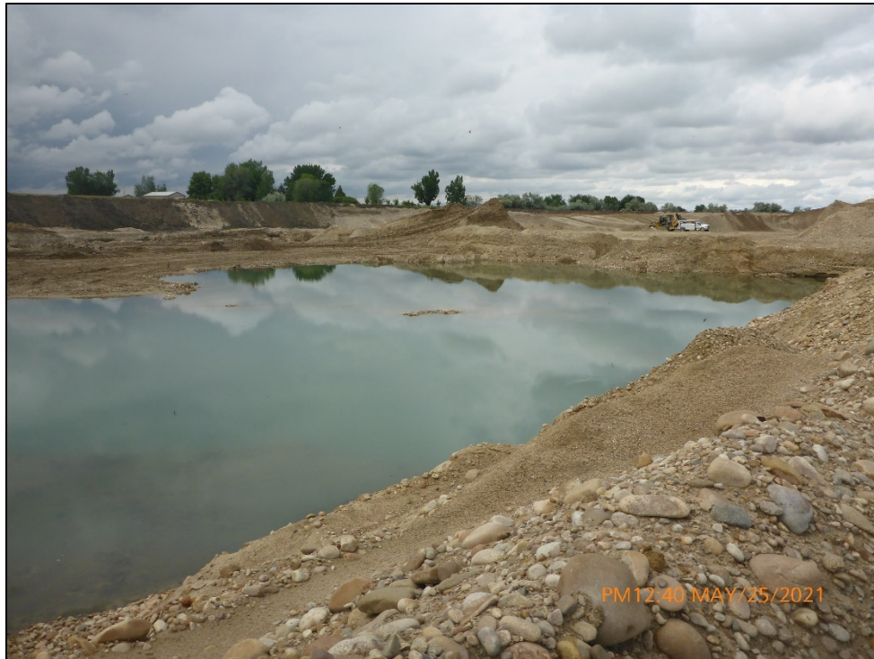
Photograph 3. View, facing southwest, of the low point in the pit area which Mr. Kalmbach identified as a groundwater accumulation area and which the SWPPP site map identifies as Sediment Pond ( refer to Exhibit 3 ).
