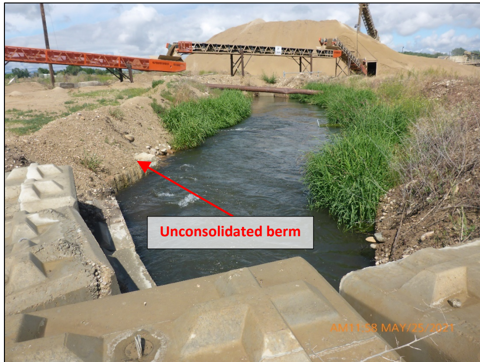
Photograph 11. View, facing west (downstream), of the tributary of the Center Point Canal that flows from east to west through the Facility. The Facility does not have outfalls that discharge into this waterbody. Note the unconsolidated soil berm adjacent to the canal.
