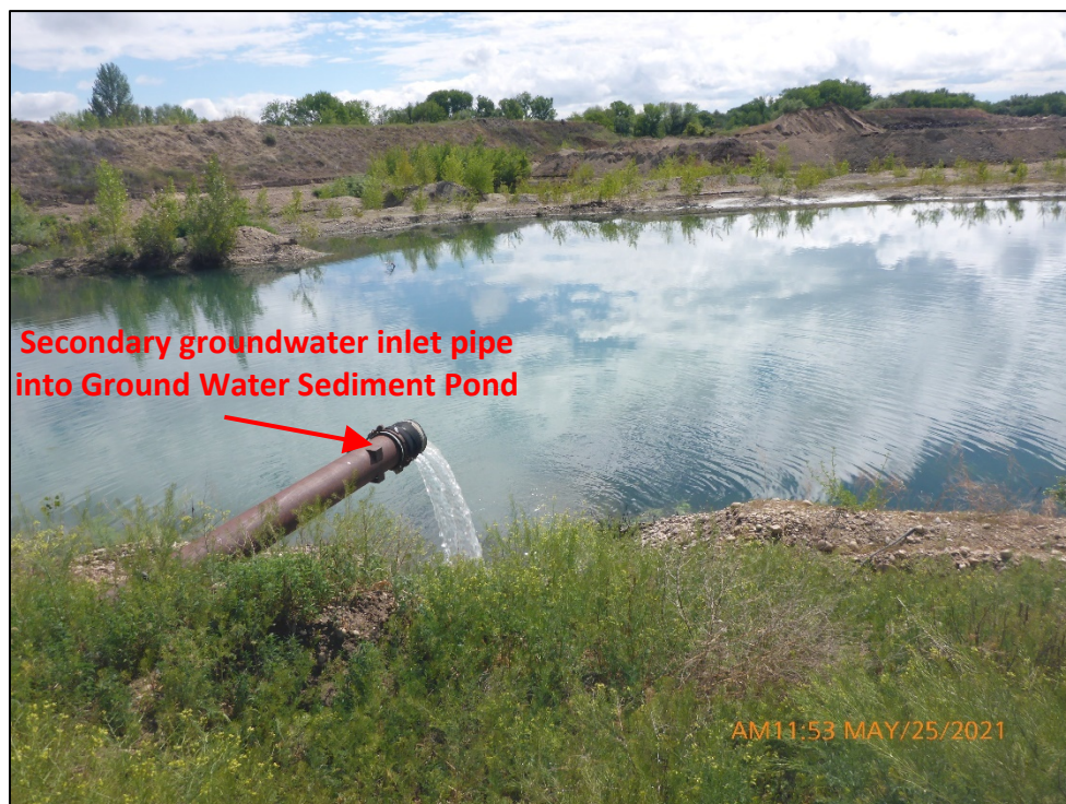
Photograph 8. View of the secondary inlet pipe (during wet season) into the Ground Water Sediment Pond.
