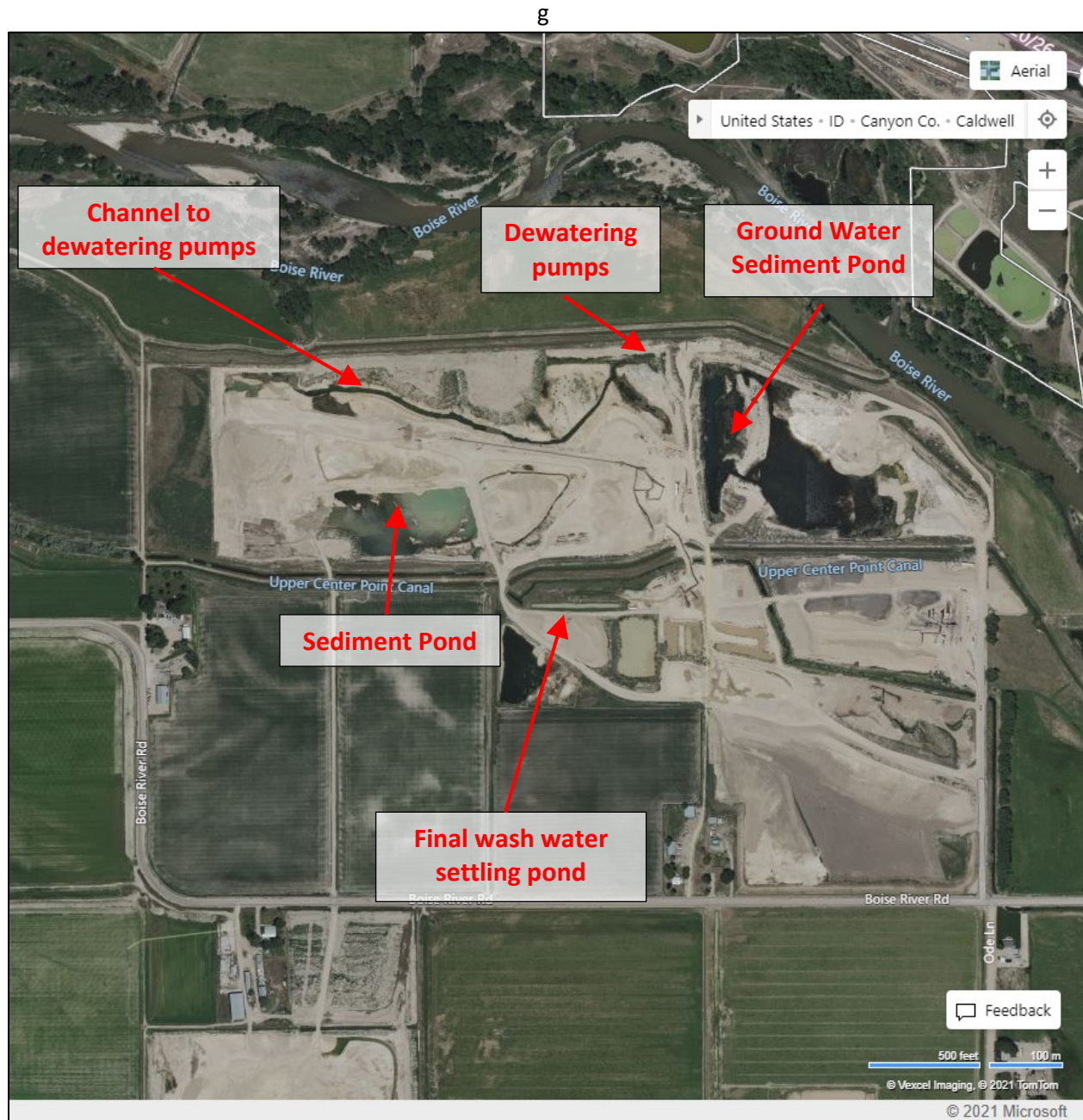
Exhibit 2. Bing Map of the Facility (imagery undated). This aerial imagery shows the expansion of the mining pit, the Sediment Pond, as well as the groundwater conveyance channel that leads to the dewatering pumps which pump to the Ground Water Sediment Pond.
