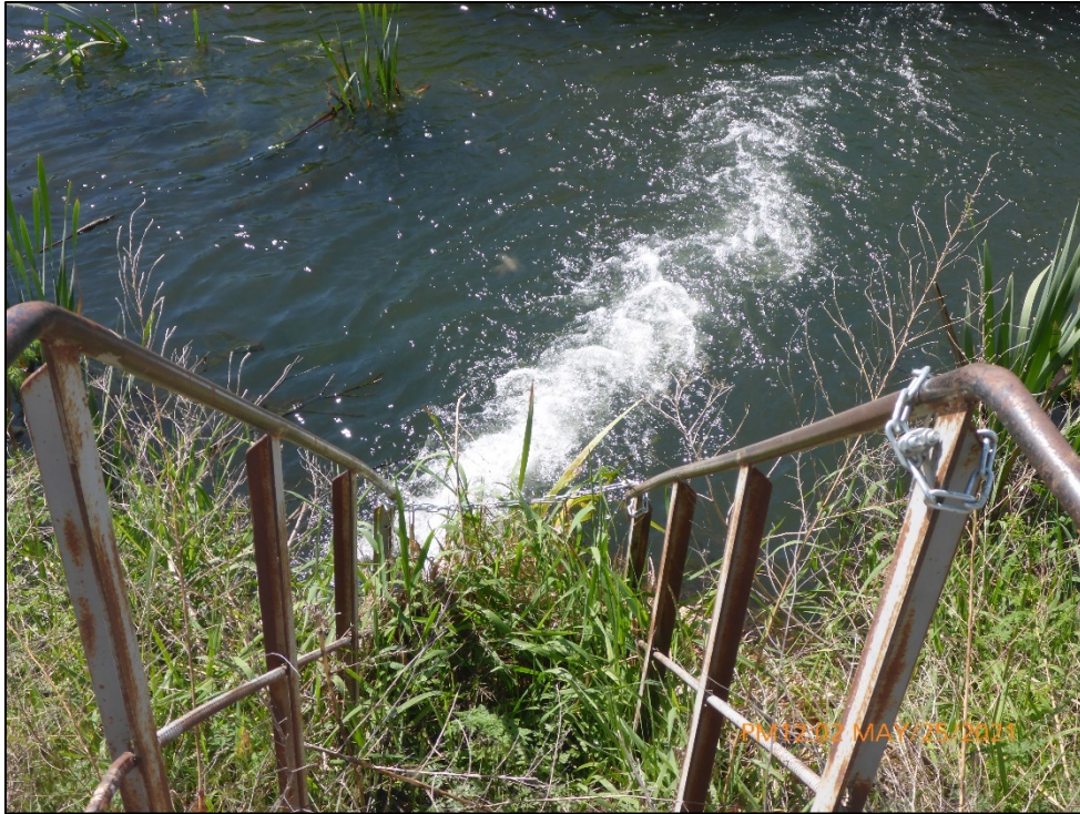
Photograph 13. Additional view of the Facility's main discharge point from the Ground Water Sediment Pond into the unnamed irrigation ditch. The stairs provide access for NPDES compliance sampling.
