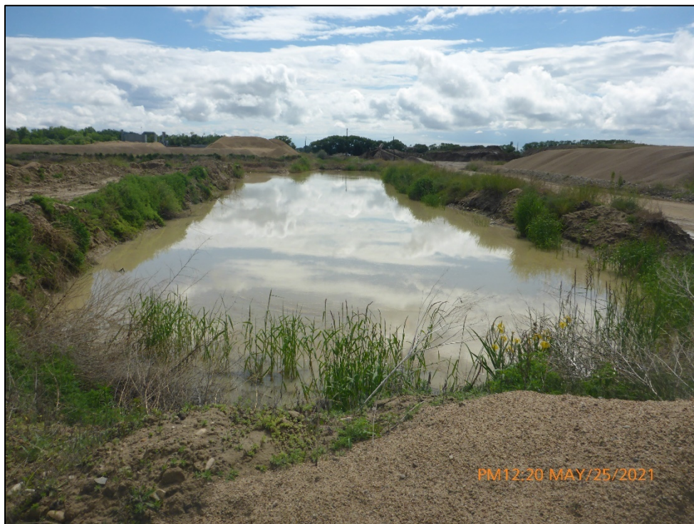
Photograph 18. View, facing east, of the second wash water settling pond.
