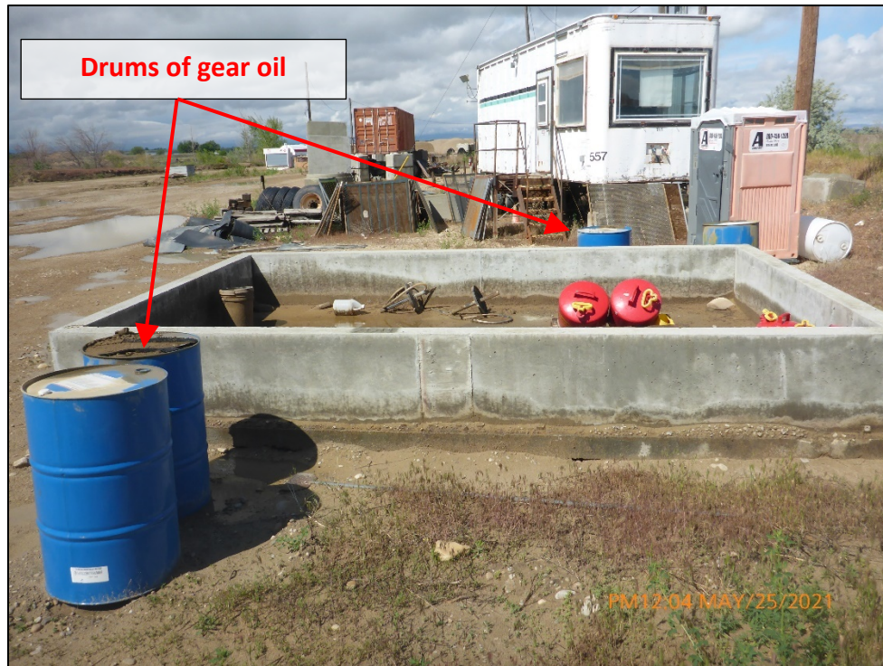
Photograph 25. View of the secondary containment structure for petroleum product storage near the aggregate wash plant. Four drums of gear oil, two empty drums and two containing product, were stored outside of the containment structure.
