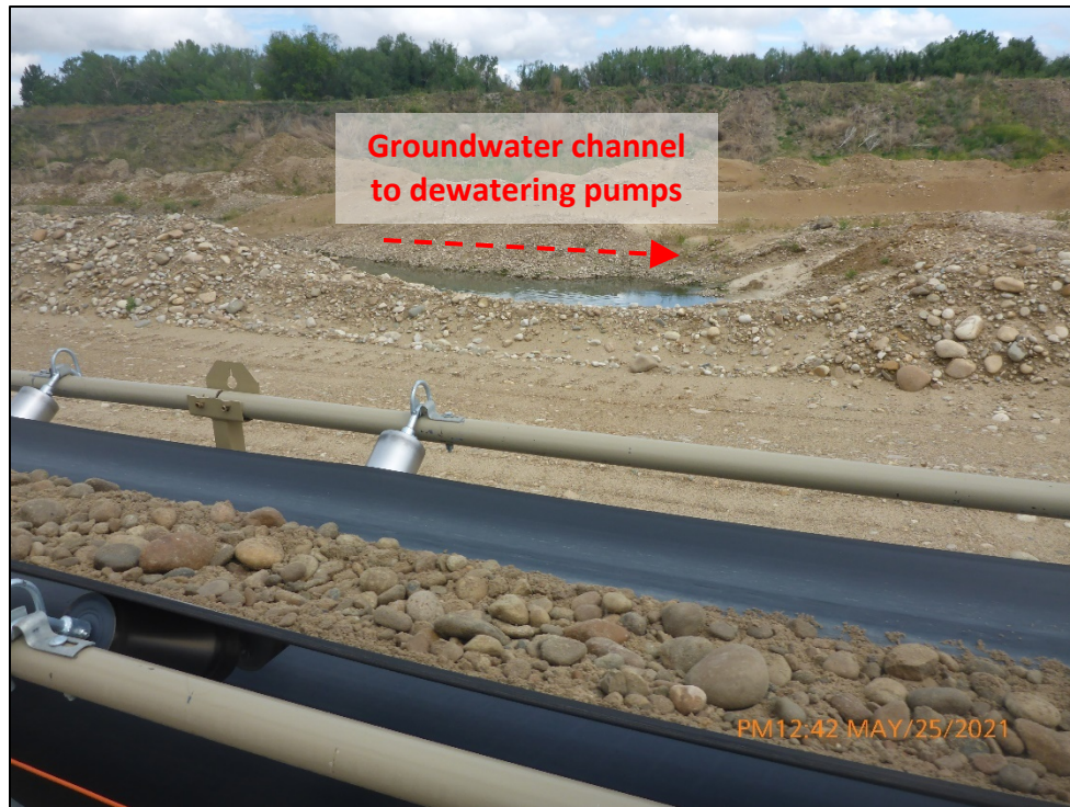
Photograph 5. View, facing north, of the approximate location where groundwater from the Sediment Pond is piped north under the main pit access road and aggregate conveyor into the channel that flows east to the dewatering pumps shown in Photograph 5.
