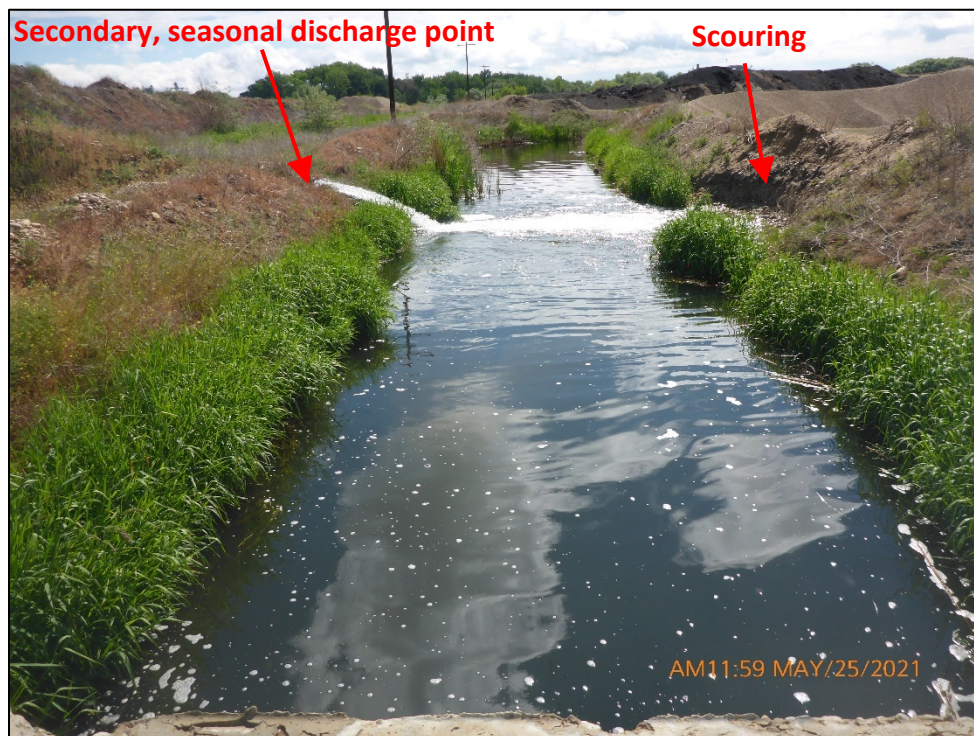
Photograph 14. View, facing east, of the Facility's secondary, seasonal discharge point from the Ground Water Sediment Pond into the unnamed irrigation ditch. Note the scouring on the embankment of the ditch adjacent to the discharge pipe.
