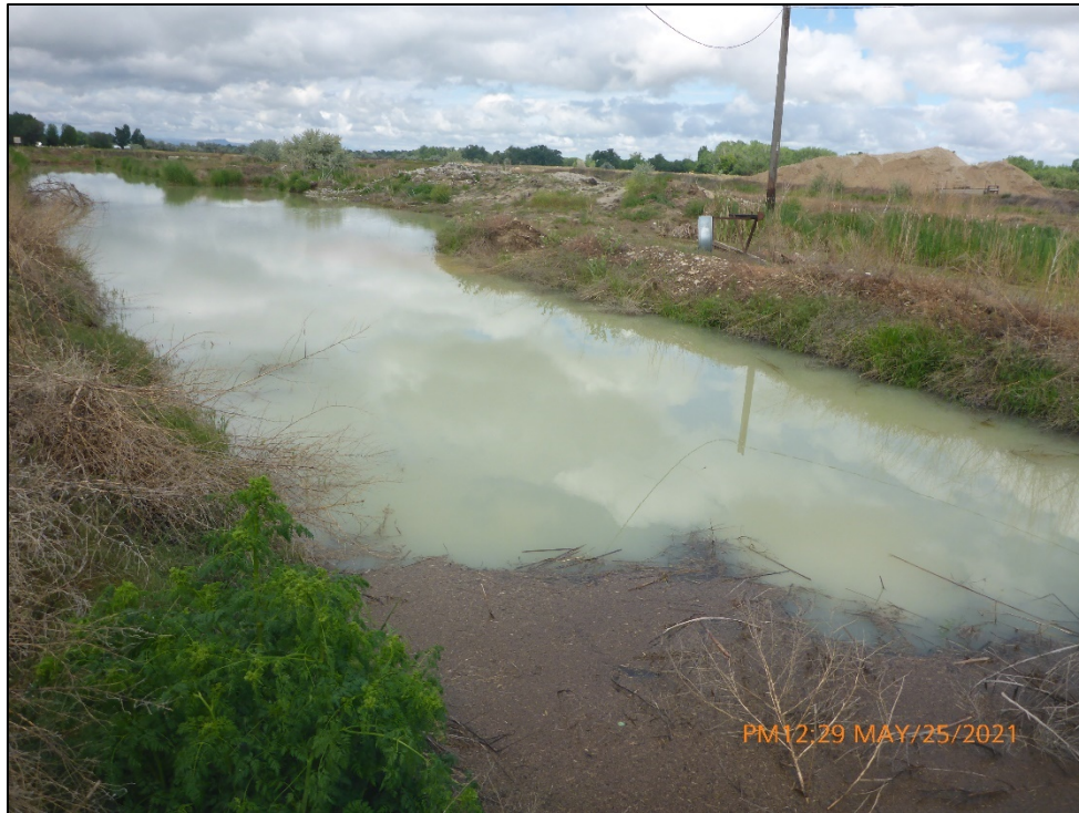
Photograph 21. View of the sixth and final wash water settling pond. Mr. Kalmbach stated that this pond does not discharge offsite. Freeboard in this basin appeared sufficient and the downgradient berm was intact and vegetated.
