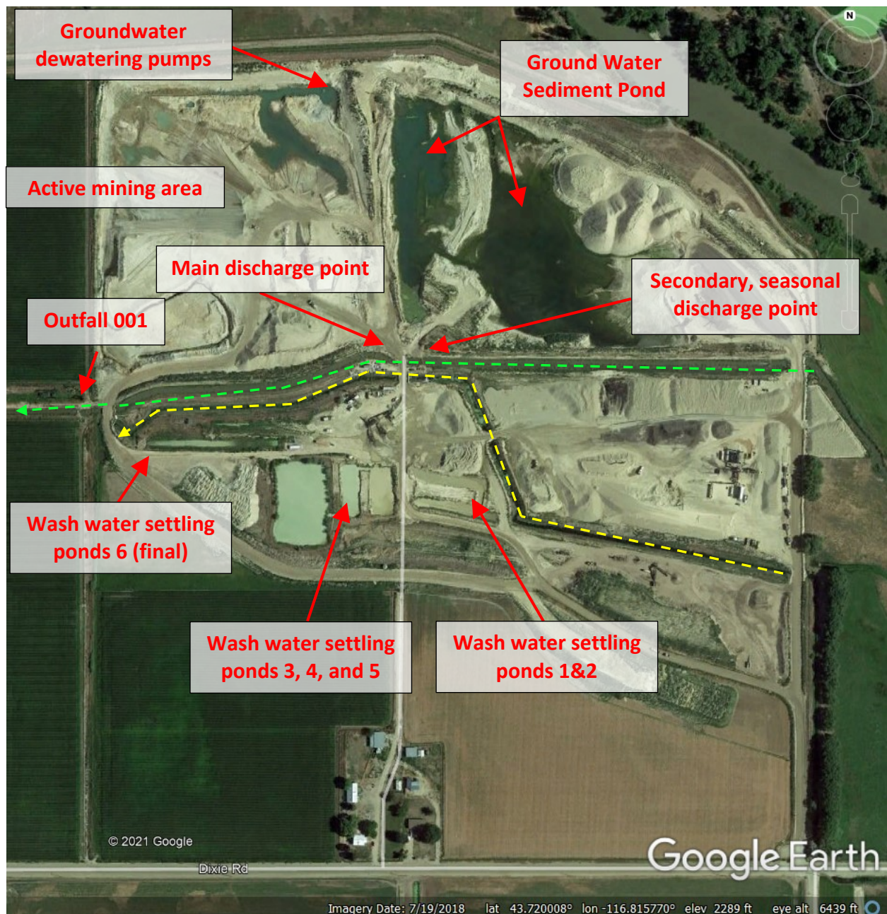
Exhibit 1. Google Earth Pro image of the Facility (imagery date: 7/19/2018). Facility features and boundaries are approximated for reference. The green dotted arrow approximates the tributary of Center Point Canal, and the yellow dotted arrow approximates the unnamed irrigation ditch.
