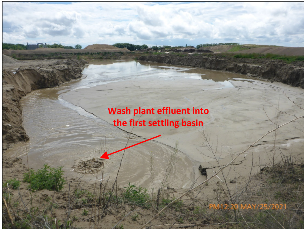
Photograph 17. View, facing southeast, of the aggregate wash water discharge point into the first of six onsite wash water settling ponds.
