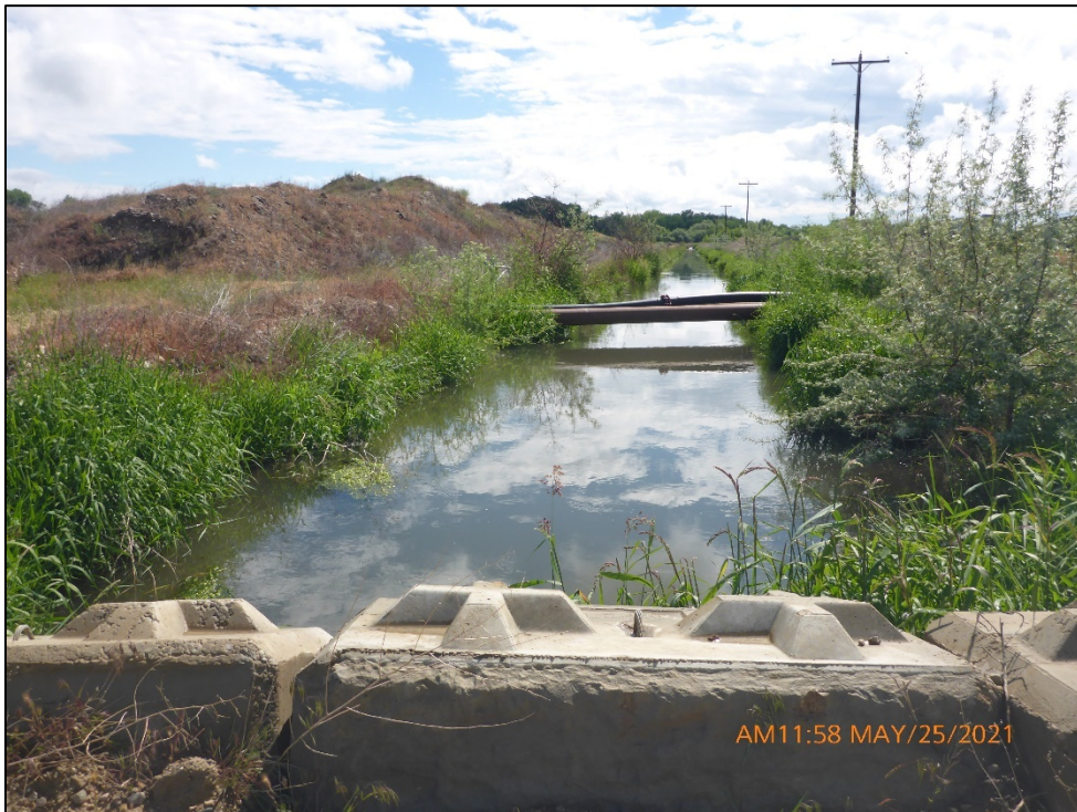
Photograph 10. View, facing east (upstream), of the tributary of the Center Point Canal that flows from east to west through the Facility. The Facility does not have outfalls that discharge into this waterbody.
