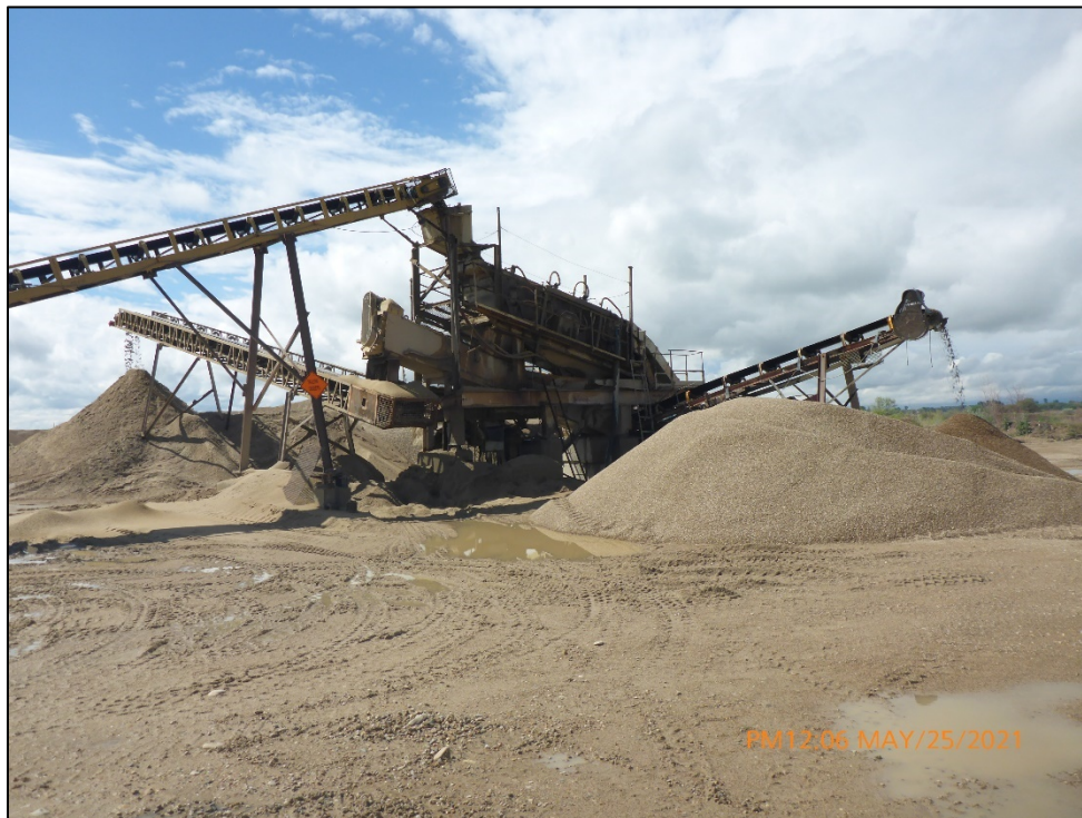
Photograph 16. View of the aggregate wash plant, which was operating at the time of the inspection.
