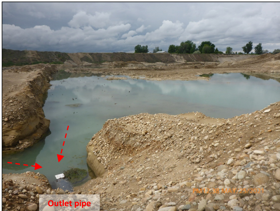
Photograph 4. Additional view, facing southwest, of the Sediment Pond and exposed groundwater shown in Photographs 2 and 3. Note the outlet pipe which conveys groundwater north, into a channel, and ultimately to the dewatering pumps shown in Photograph 5 and 6.
