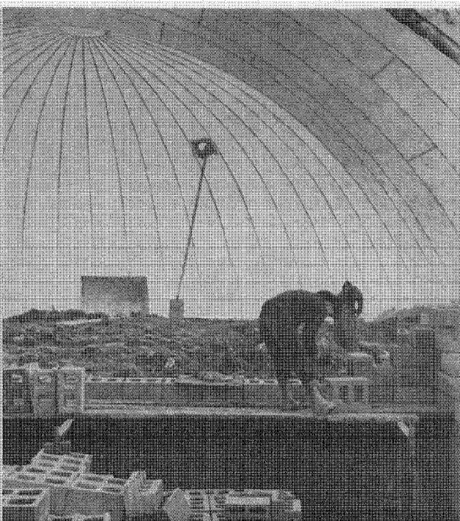
Protected from weather, masons work at night laying foundation, keeping fantastic winter schedule of 21 days per house.
