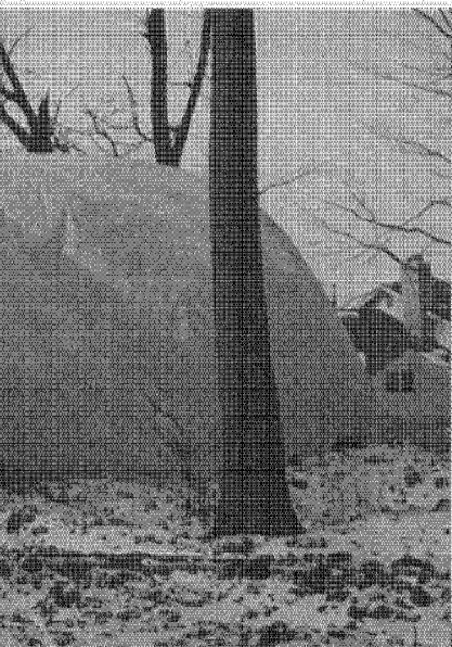
On the way up, nylon air shelter developed by homebuilder Robert Brown covers house site and building materials.
