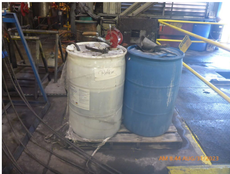
Photograph 1. Chemical storage drums lacking secondary containment.
