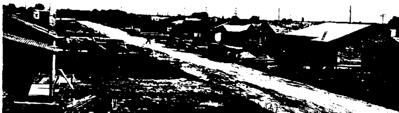
General view of the Gardner Addition in which lead plumbing predominates
