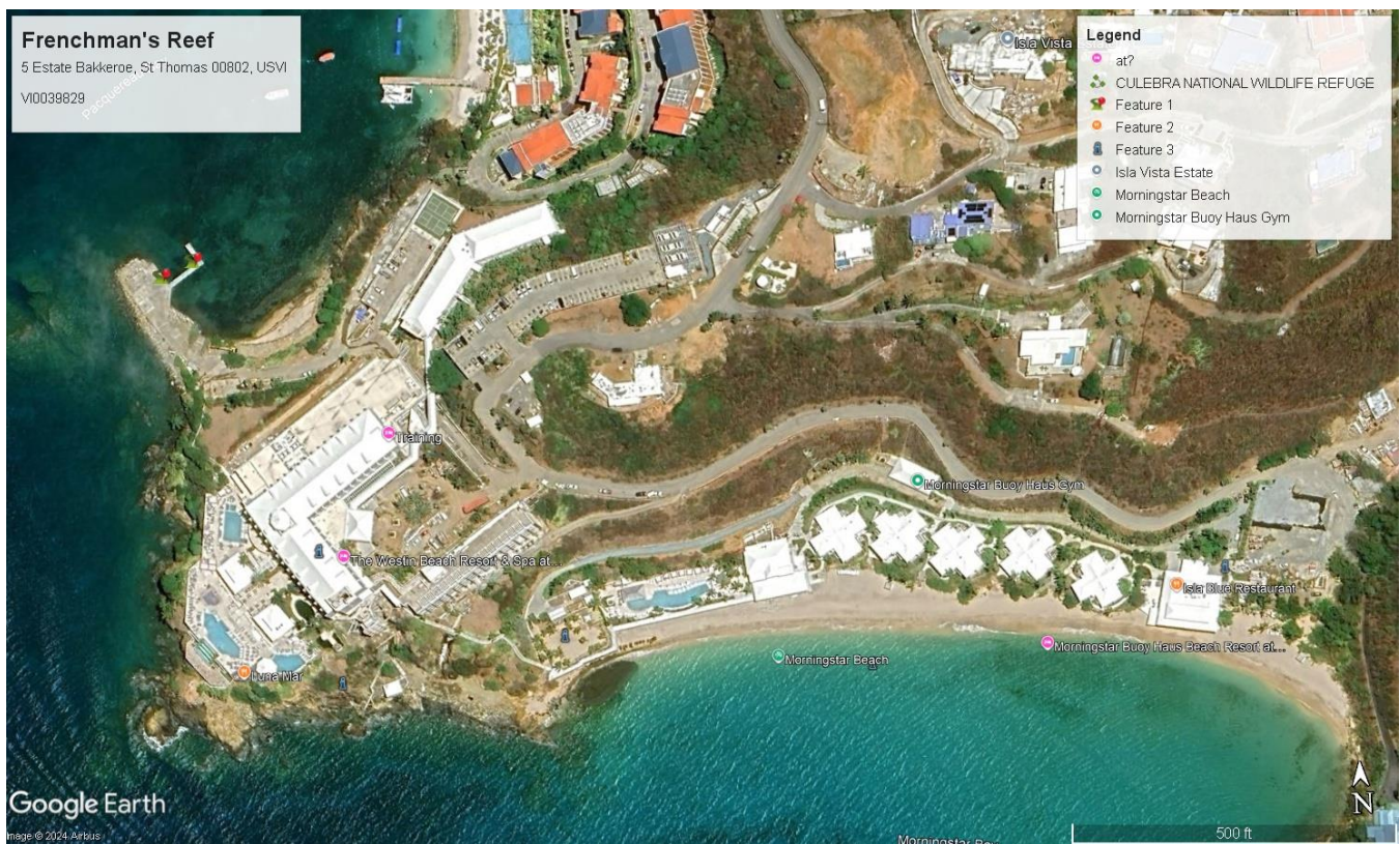
Image 1 – Aerial photograph, featuring the Frenchman’s Reef Compound 5
