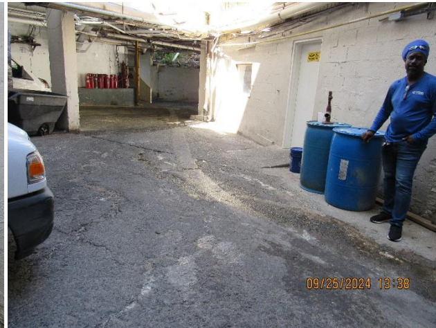
IMG 1380 -Existing stormwater flow path in LUB area, that drains down gradient towards the Back-Of House (BOH) 2 area and into stormwater catch basins just downstream.
