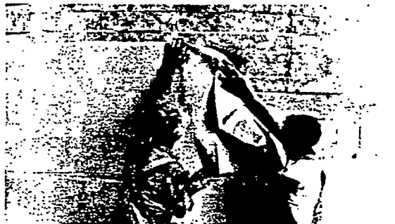
For an indoor finish on heated equipment, hydraulic setting insulating cement is used, then canvas and a coat of resin base adhesive.
