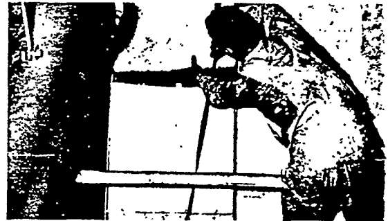
After any necessary cutting and shaping, Fiberglas Equipment Insulation can be banded in place or held with welded pins or studs.
