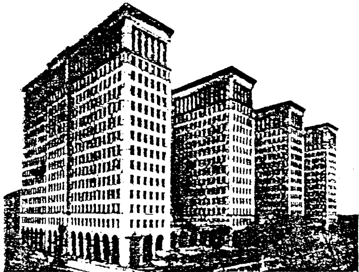
OFFICE BUILDING—PAINTED WITH DU PONT PRODUCTS
