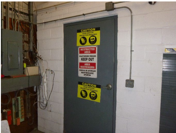
Photograph 9: Containment Room in Building 1.
