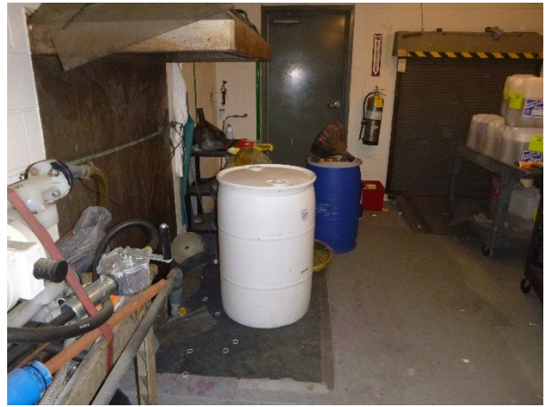
Photograph 10: Containment Room in Building 1.
