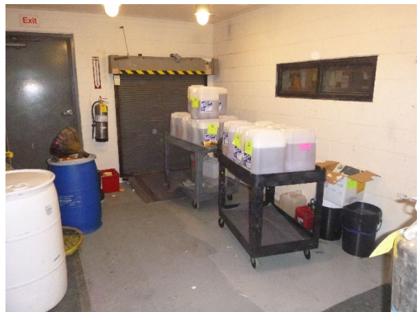
Photograph 11: Containment Room in Building 1.
