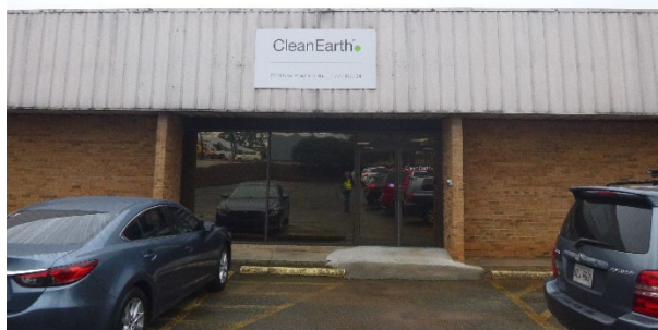
Photograph 1: Exterior of Building 1.
