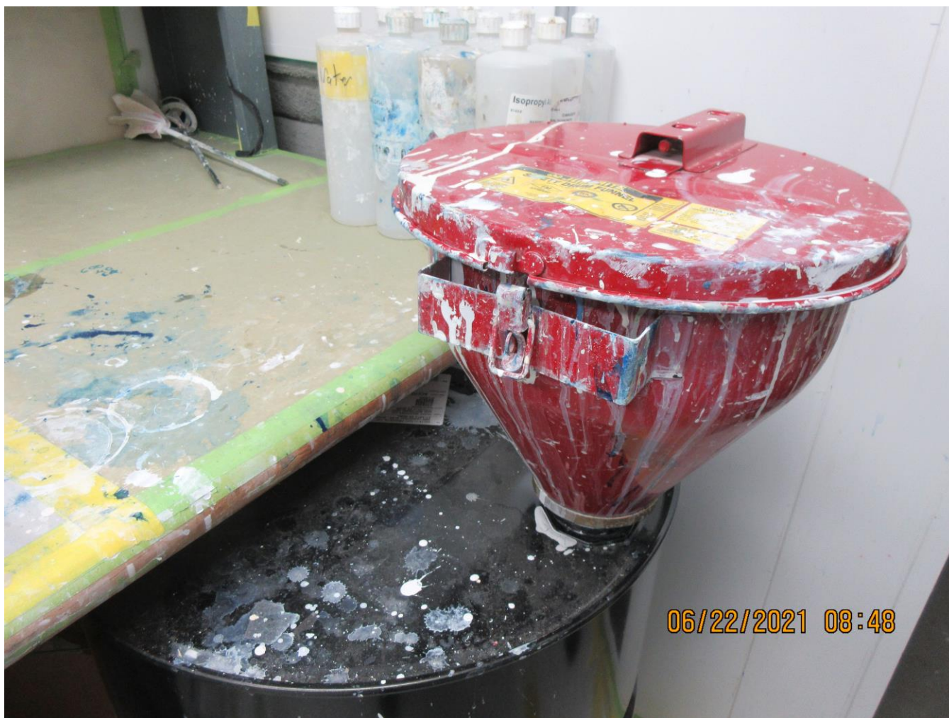
Photo 12 – Hazardous Waste Container in Paint Booth on Composites Site
