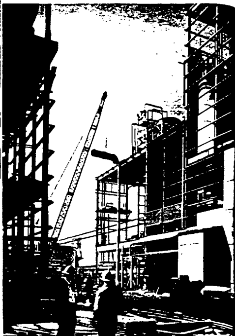
A huge crane hoists equipment into the salt processing wing of the sodium building as it nears completion. Here, salt will be electrolytically decomposed into its elements, sodium and chlorine. At left is chlorine building.
