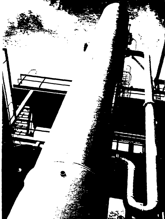
Like a giant cannon, the tower in the ethyl chloride area at the new Houston plant casts an impressive figure against the Texas sky.
