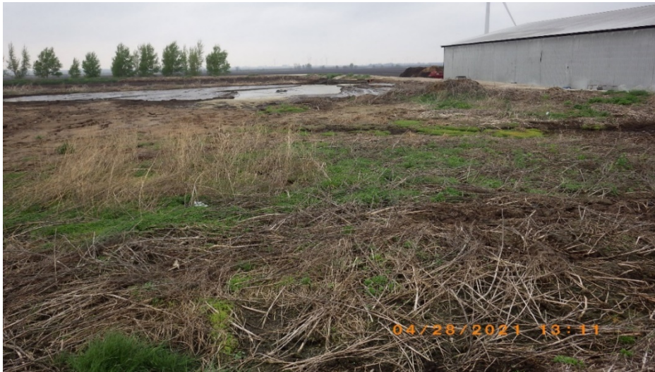
Photo Number: RIMG0176 Description: The 1 st Stage Lagoon and Commodity Shed. Location: Southwest corner of the Commodity Shed. 40.485617, -87.496863 Facing: North. Date/Time: 4/28/2021 1:11 p.m.
