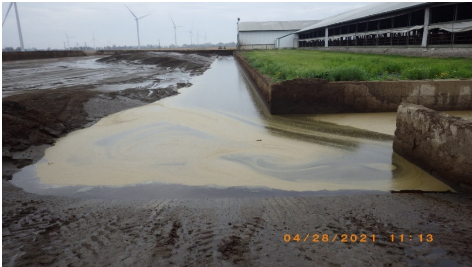
Photo Number: RIMG0095 Description: Sand Separation Lane which is pumped into the 1 st Stage Lagoon. Location: In the Solid and Sand Stacking Pad area west of the Sand Separation Lane. 40.487351, -87.495501 Facing: East. Date/Time: 4/28/2021/ 11:11 a.m.
