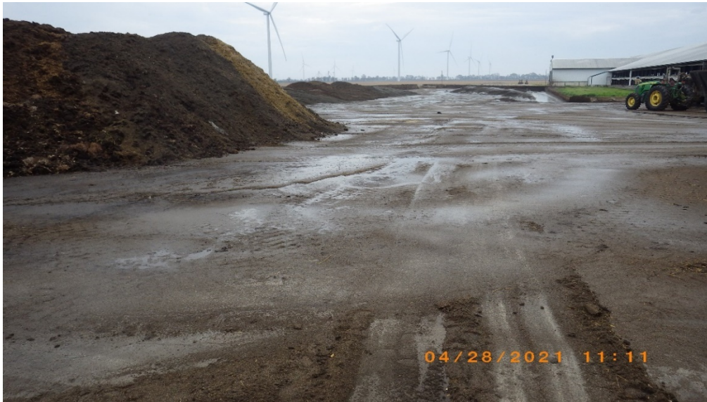
Photo Number: RIMG0094 Description: Solid and Sand Stacking Pad. Location: West side of the Solid and Sand Stacking Pad. 40.487473, -87.495233 Facing: East. Date/Time: 4/28/2021/ 11:09 a.m.
