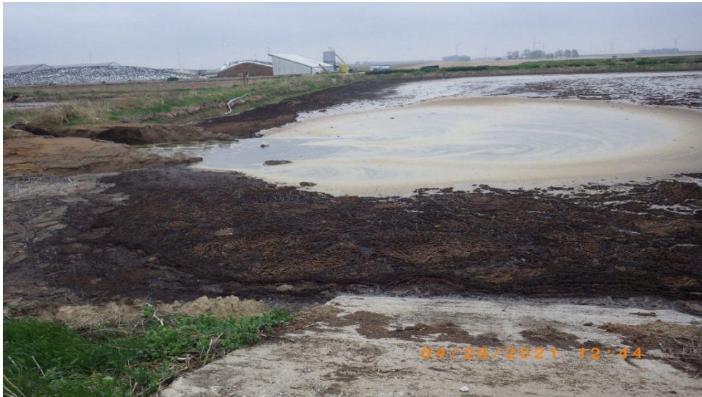
Photo Number: RIMG0154 Description: Access pad to the 3 rd Stage Lagoon. Location: North side of the 3 rd Stage Lagoon. 40.48688, -87.499627 Facing: West. Date/Time: 4/28/2021 12:44 p.m.
