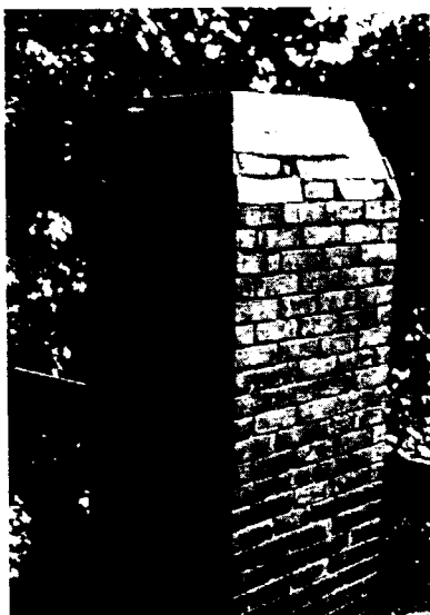
Two views showing the deterioration of the chimneys due to attacks by the weather
