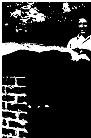
Views showing rebuilt chimney, without lead cap, dressing the lead over the chimney cap, and the finished lead chimney cap in place, adequate protection against deterioration
