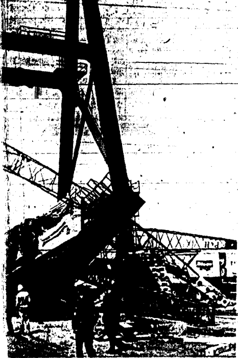
INJURED IN COLLAPSE OF 80-TON CRANE s estimated at between $100,000 and $250,000
