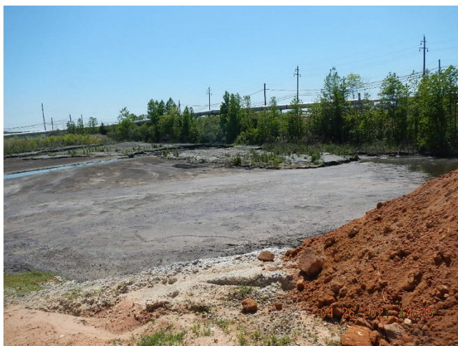
Photo 5. EQ Basin, west/influent side.
