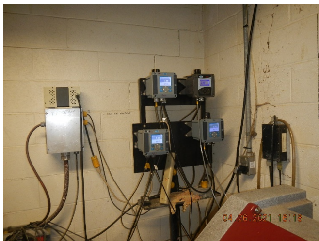
Photo 15. Dissolved Oxygen and pH meter display. Post-aeration Basin equipment room.
