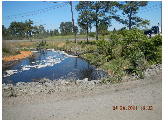
Photo 8. Inlet Ditch from EQ Basin outlet.
