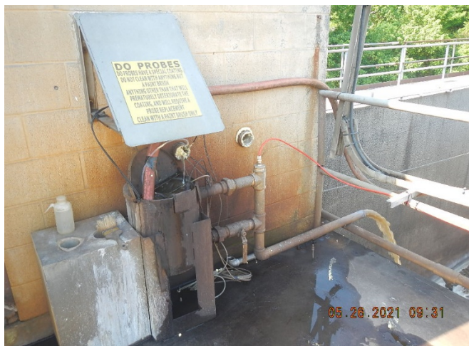
Photo 17. Post-aeration Basin. Sampling box observed on May 26 th .
