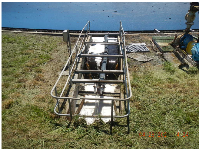
Photo 3. Outfall 01A, domestic wastewater outfall.
