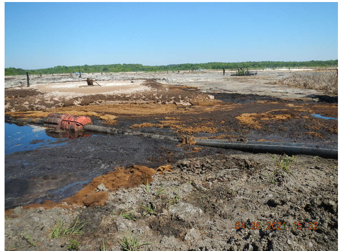
Photo 10. ASB northwest end looking south-southeast. The HDPE pipe is a 10" inlet pipe used to discharge foul condensate directly into the ASB from the process area.
