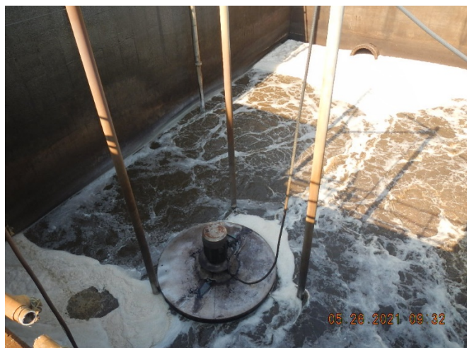
Photo 14. Post-aeration Basin interior, May 26 th .
