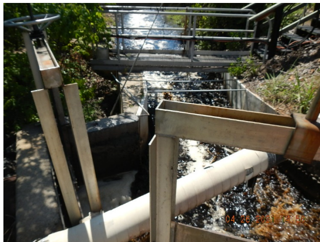
Photo 4. Open channel ditch directing flow from the Primary Clarifier to the EQ Basin and EQ Basin Bypass Pipe inlet.
