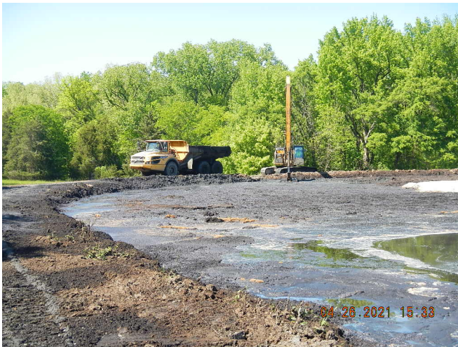
Photo 9. ASB northwest end new the Inlet Ditch. Excavator dredging operations in progress.
