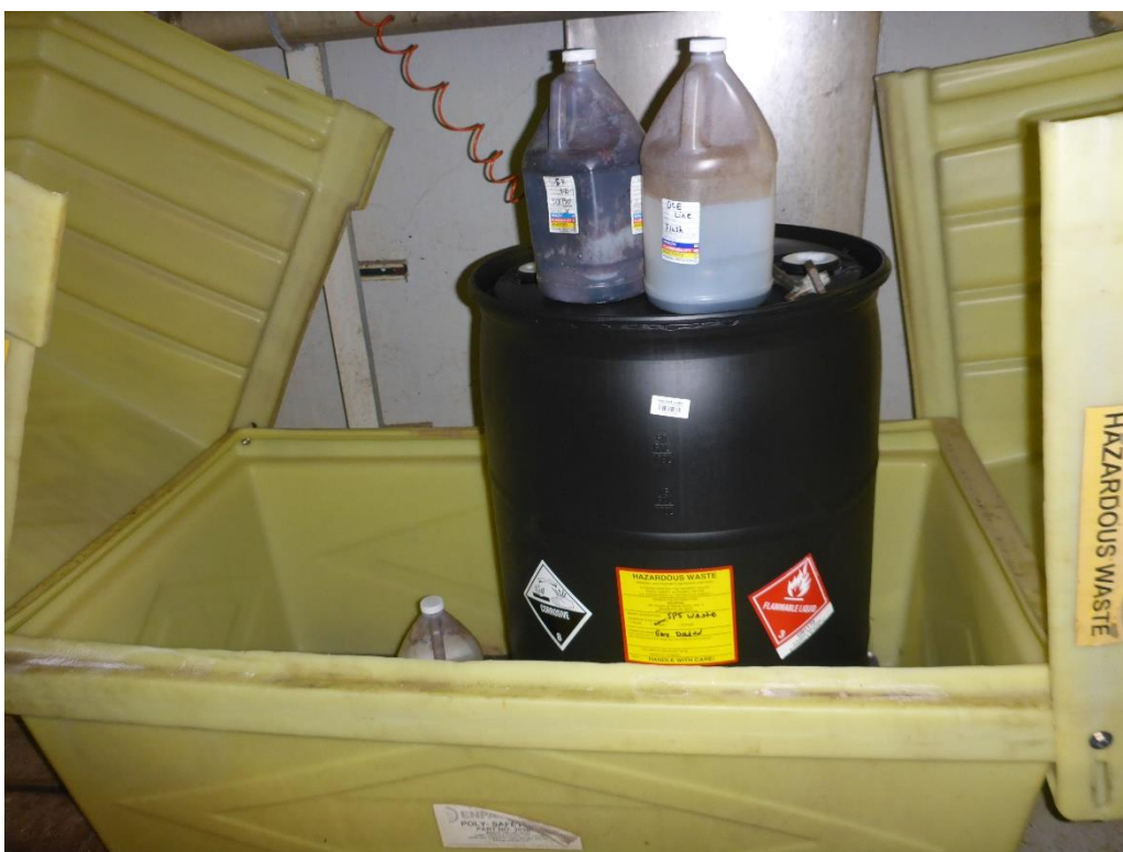
Photo 5: Two one-gallon jugs inside the locked, plastic clam-shell secondary containment unit at SAA #4. The jugs were each labeled DCE Line Flush and identified with a Hazcom label. One jug was dated 03/21/2019. The drum was labeled hazardous waste and identified with flammable liquid and corrosive DOT hazard placards, but it was not identified with a toxic DOT hazard placard.
