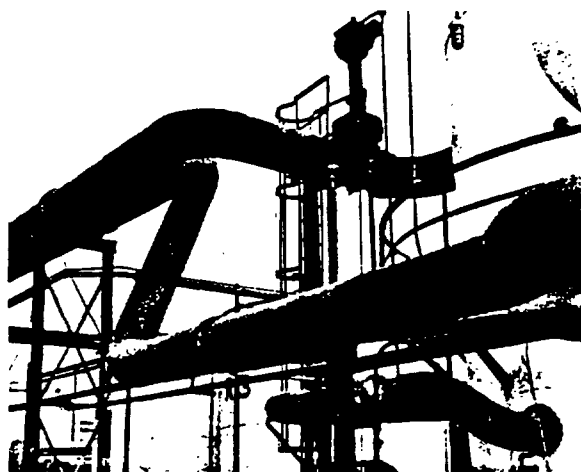
The piping at this large Illinois refinery is protected by UNIBESTOS. Note the ease with which the fabricated sections of UNIBESTOS accommodate the sharp bends of the piping.
