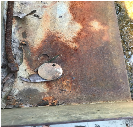
Picture 20: Tags associated with the Ancillary Equipment were not clear and visible and Signs of Paint peeling (Tank #1)
