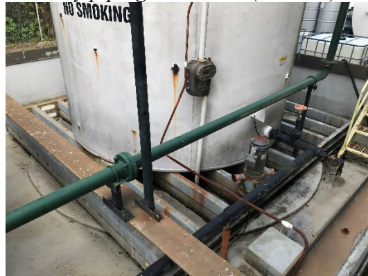
Picture 23: Empty Vertical Mounted Tank in Secondary Containment no longer in service (Tank #2)
