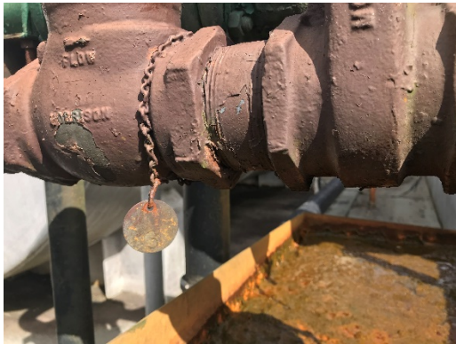
Picture 20: Tags associated with the Ancillary Equipment were not clear and visible and Signs of Paint peeling (Tank #1)
