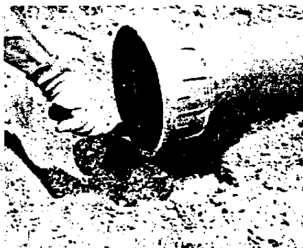
Buttering the shoulder at the base of the bell with FURATHANE Mortar. Do not butter the sides of the bell.
