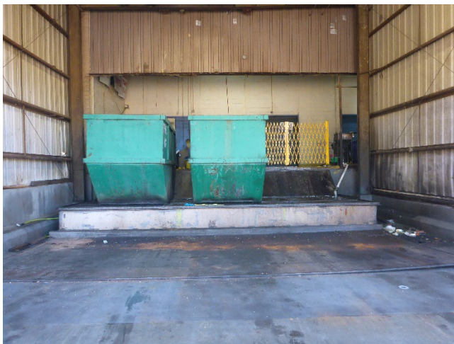
Photo 15: Two of three large hoppers staged above the 2,500-gallon metal fabricated storage tank at the Chip Dock. The funnel and PVC pipe shown in Photo 17 can be seen to the right at the far side of the tank. The blind sump shown in Photo 18 can be seen to the right at the near side of the tank.
