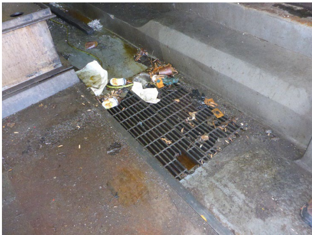
Photo 18: Blind sump located next to the 2,500-gallon metal fabricated storage tank at the Chip Dock. Facility personnel stated that this sump is connected to the sump observed inside the room with the 2,000-gallon storage tank, but that liquids do not drain from the sumps. Instead, when the transporter comes to transport liquids from the 2,000-gallon and 2,500-gallon tanks, liquids are also pumped from the sumps and shipped with the tank contents.
