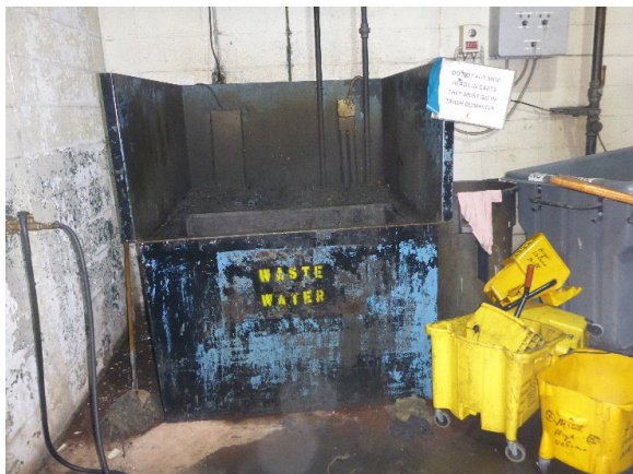
Photo 9: Large open vat labeled “waste water” in the Chip Dock Area. Dirty mop water, including the dirty mop water that is accumulated in the 110-gallon container shown in Photo 2, is poured into this vat. The dirty mop water is then transferred into a 2,000-gallon vertical storage tank, which is located on the other side of the cinderblock wall behind the vat.
