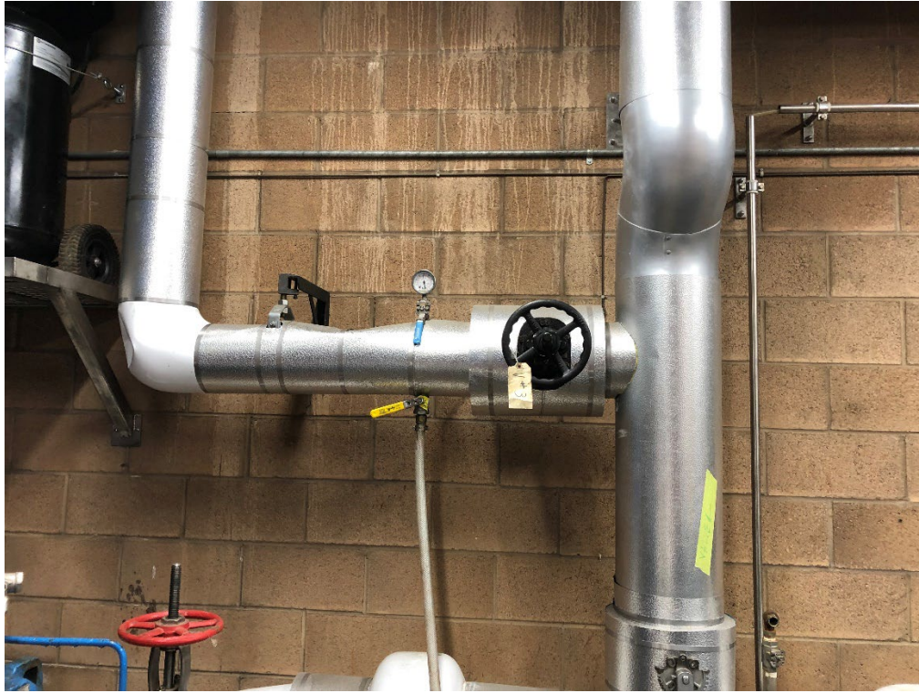
Photo #3. A grab sample was collected of the groundwater at the influent sample point.
