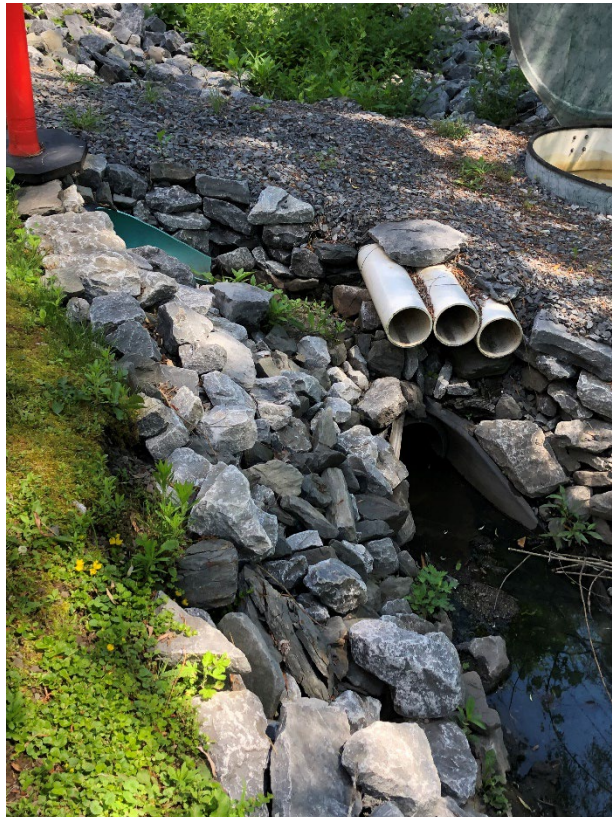
Photo #4. No discharge was observed from the stormwater outfalls during the inspection.
