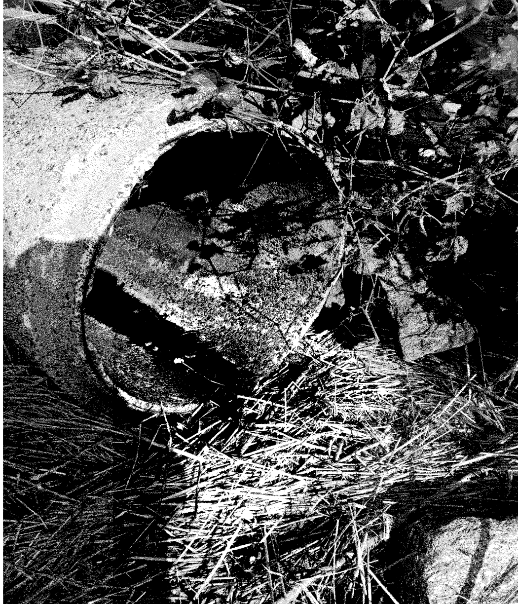
Photo 2: Beacon1 (photo taken 10/22/2024 at approx. 10:21 Outfall located near 2 Seabright Ave, discharging into the Long Island Sound. Sample point is indicated by a red X. (Note1: Time stamp on photo is incorrect) (Note 2: Not enough flow to collect adequate sample volume for PCP, enterococcus analysis, conductivity, salinity, and temperature. Only enough discharge to analyze for ammonia, surfactants, and total chlorine.)
