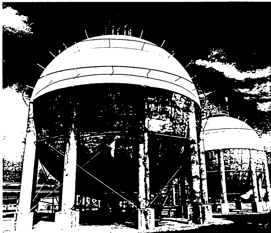
Storage spheres at PPG's Lake Charles, Louisiana plant hold thousands of gallons each of liquid vinyl chloride monomer under pressure
