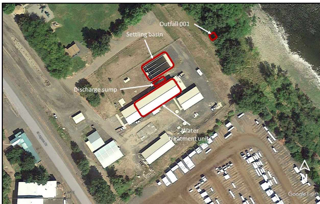
Figure A-1. Satellite imagery of the facility with relevant areas and assets outlined in red.
