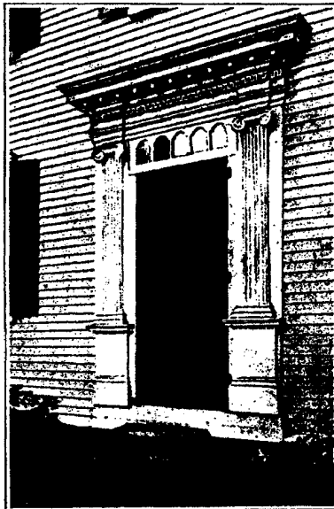
Detail of doorway of the Stebbins house. Although more than 150 years old, every piece of the architectural detail is preserved perfectly. Yet the stone used as a step has been gradually destroyed by the elements until it was necessary to place a small stone on top of the original.
