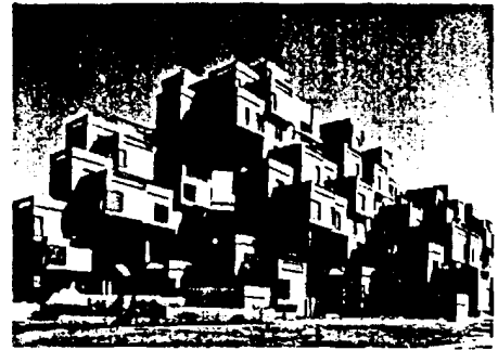
HABITAT 67 incorporates many new architectural designs, including prefabricated bathrooms of Glidden's polyester resins finished with Gel-Kote.
