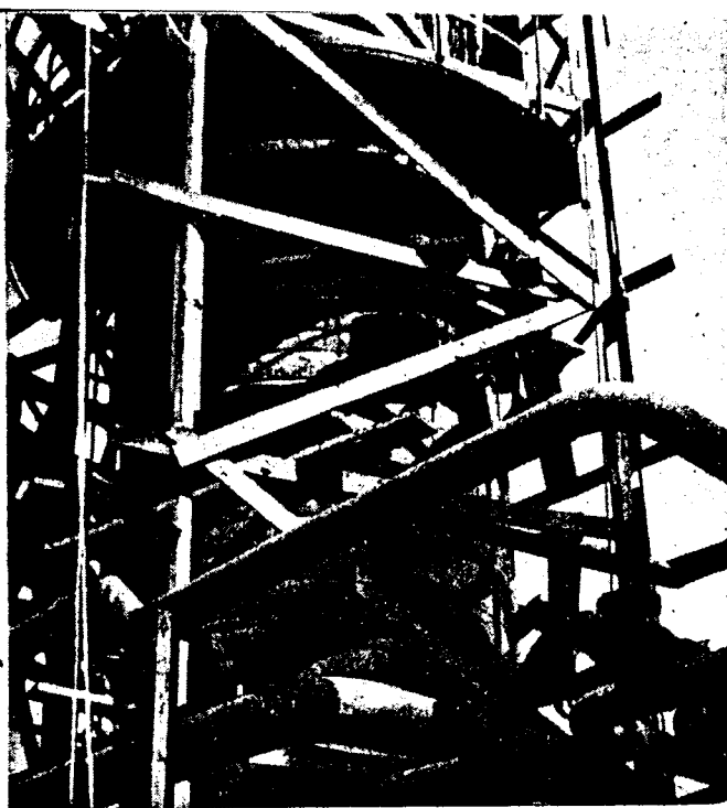
Mineral wool blankets banded in place on fractionating tower.
