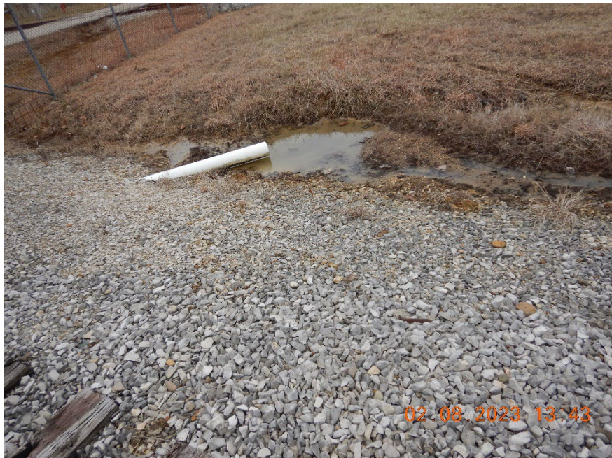
37: DSCN1163 Description: Stormwater Outfall 021 Location: Building 104 Area Camera Direction: North Date/Time: 10/12/22, 1:37 p.m.
