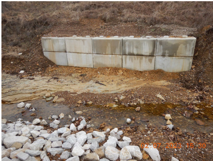
17: DSCN1143 Description: Concrete blocks to combat erosion at stormwater trench from burn pits Location: ABG Camera Direction: Northeast Date/Time: 2/7/23, 3:30 p.m.
