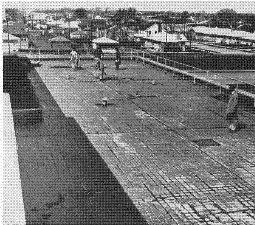
BEFORE. While this roof offers protection from weather, it has little other use. Shortage of usable space, however, has caused new duties to be assigned to
