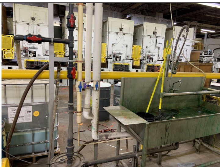
Wash station with 275-gal container for cleaner washout. Photograph 4 taken at 11:27am
