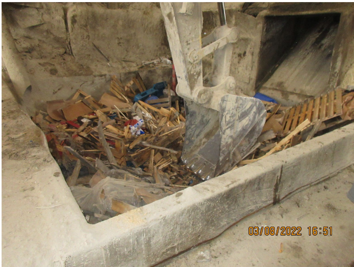
Photo 10 – Treatment Unit within Area B of Unit 207
