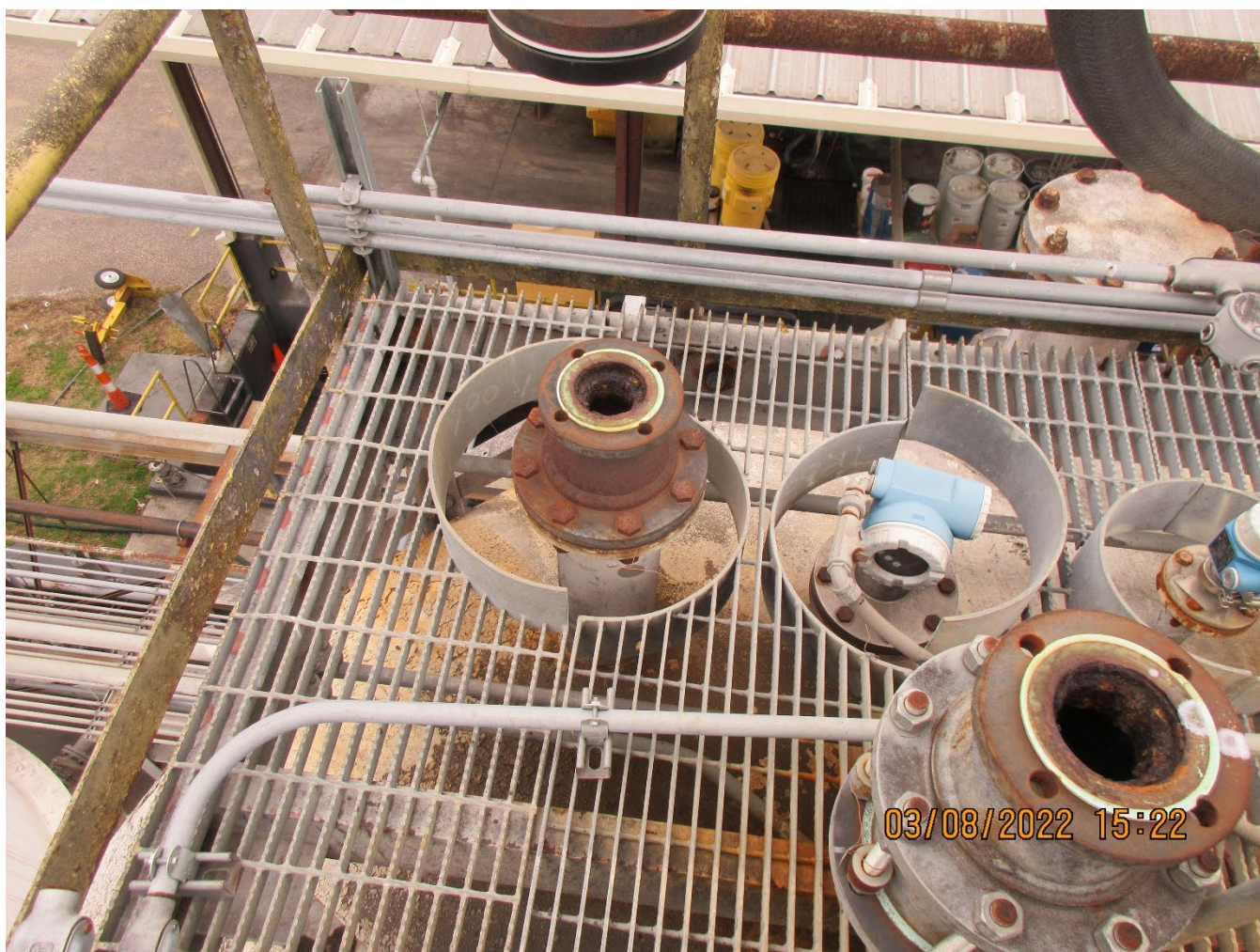
Photo 8 – Top of Tank 4. Equipment removed during repair.
