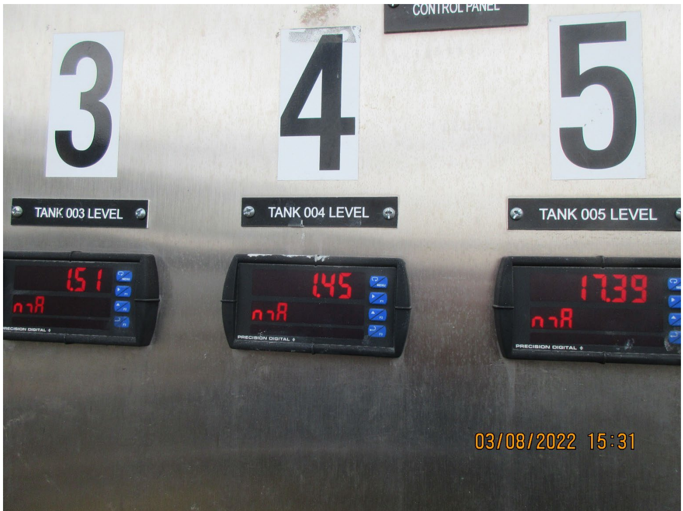
Photo 9 – Level readings for Tanks 3, 4 & 5
