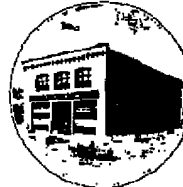
MINNEAPOLIS DEPOT WESTERN DIVISION
