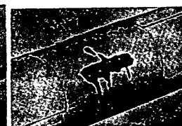
STEP FOUR Asphalt poured in slot—a perfect seal.
