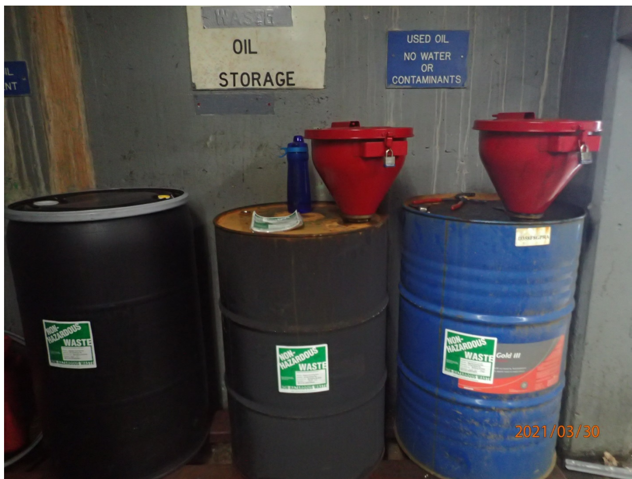
Photo 23: Three 55-gallon drums of used oil with locked funnel lid. Small bung open on one used oil drum (middle). Inside Oil Room in Magnolia Plant.
