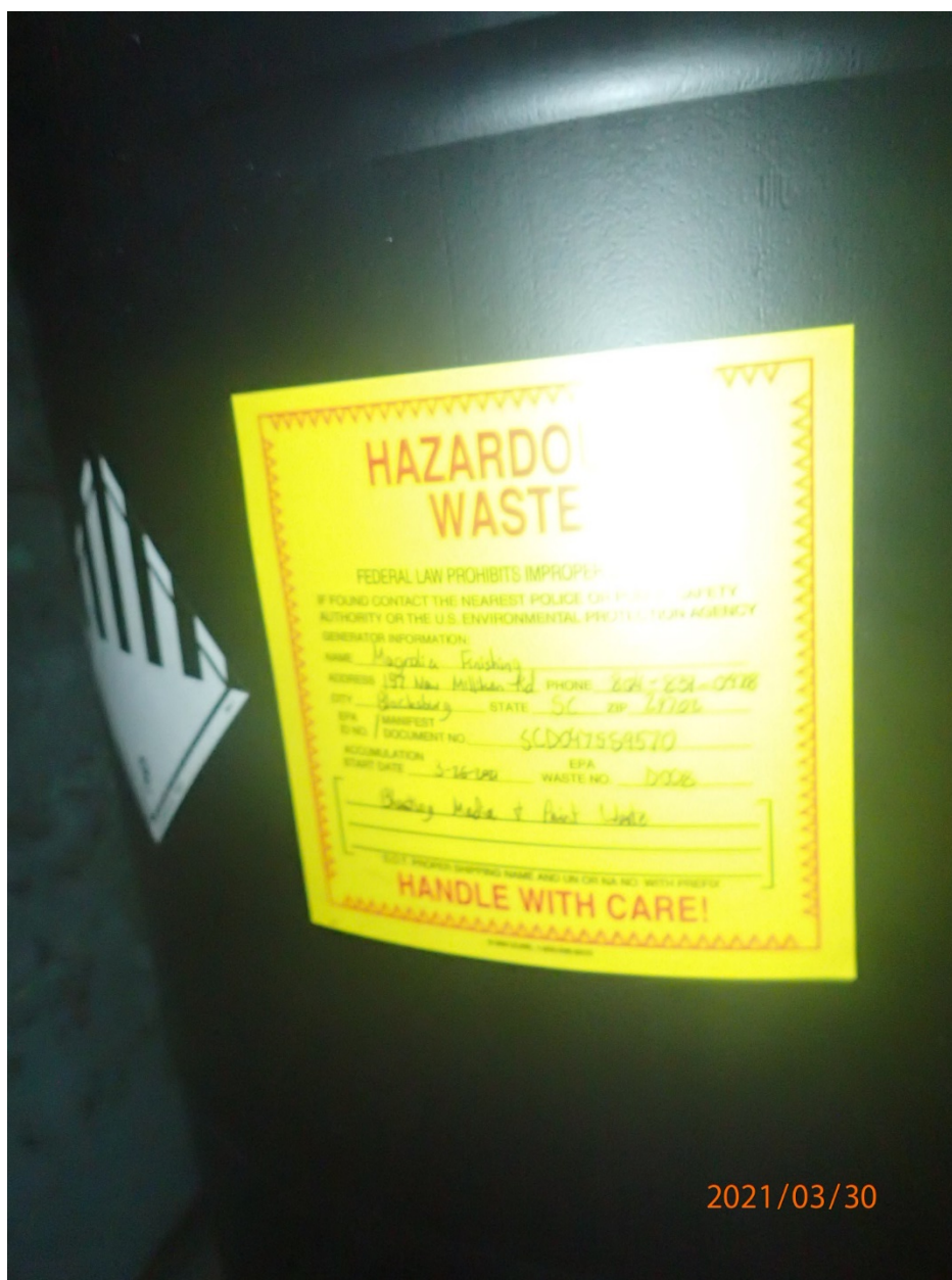
Photo 7: 55-gallon drum with label for blasting media and paint waste. Located inside Pen 1 in Magnolia Plant.
