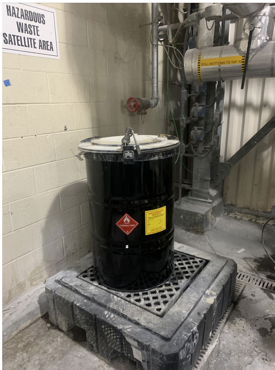
Photo 26: Photo taken by Rob Wallace, Environmental Manager at Allen Plant. AF Building. 55-gallon drum for filter bags from the recirculation line, labeled “Hazardous Waste Flammable Liquid D001”.
