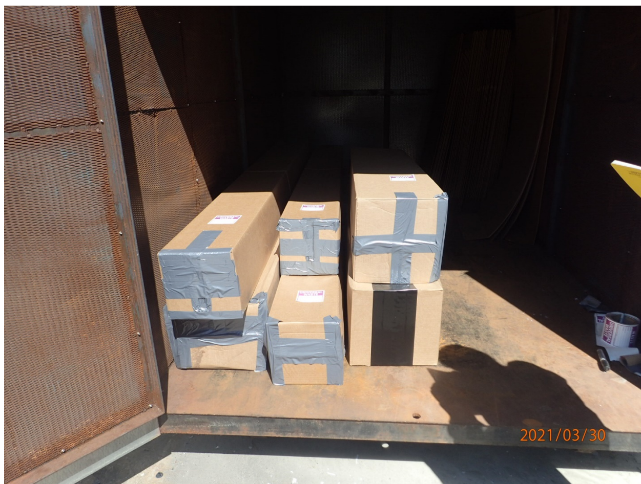
Photo 19: Storage area for Universal Waste Spent Fluorescent Bulbs. Four 8-ft boxes and two 4-ft boxes. Magnolia Plant.
