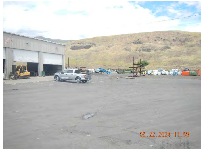
Photo #:24 (DSCN3763) Description: Facing north, photo of paved collection area for catch basin Outfall 001.
