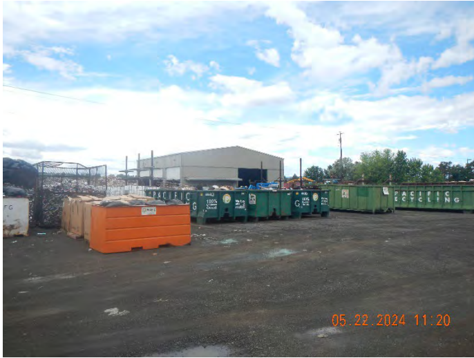
Photo #:05 (DSCN3744) Description: Facing south, photo within material storage area. Bins are delivered and stored temporarily until brought into the crushing/processing area.
