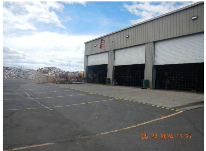
Photo #:08 (DSCN3747) Description: Facing south, photo of catch basin drainage/collection area for Outfall 001. Photo taken east of the New Steel Building.
