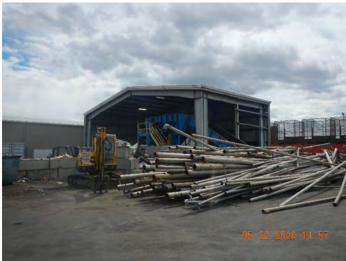
Photo #:23 (DSCN3762) Description: Facing southeast, photo of staged aluminum piping awaiting cutting. Due to length/size, piping was staged at location. Area is northeast of mixed recycling receiving area.
