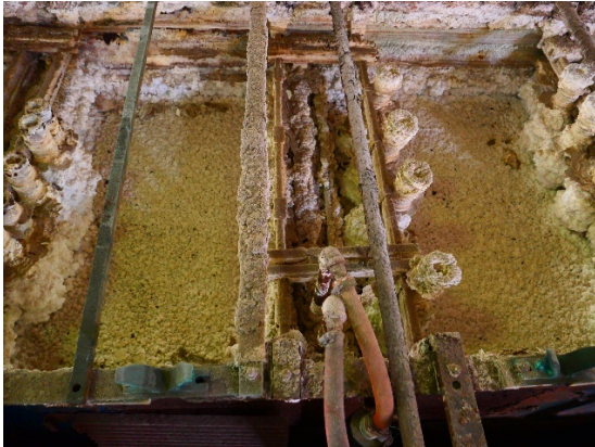
Photo #1 – Out of service zinc plating large barrel line tanks.
