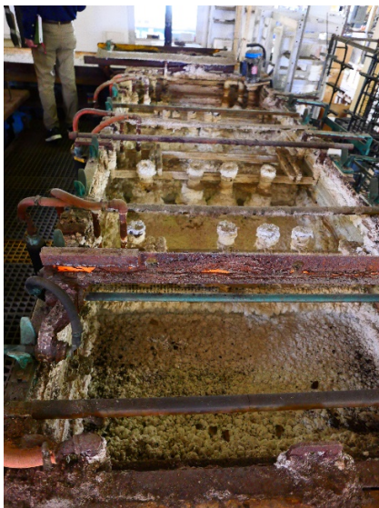
Photo #3 – Out of service zinc plating large barrel line tanks.
