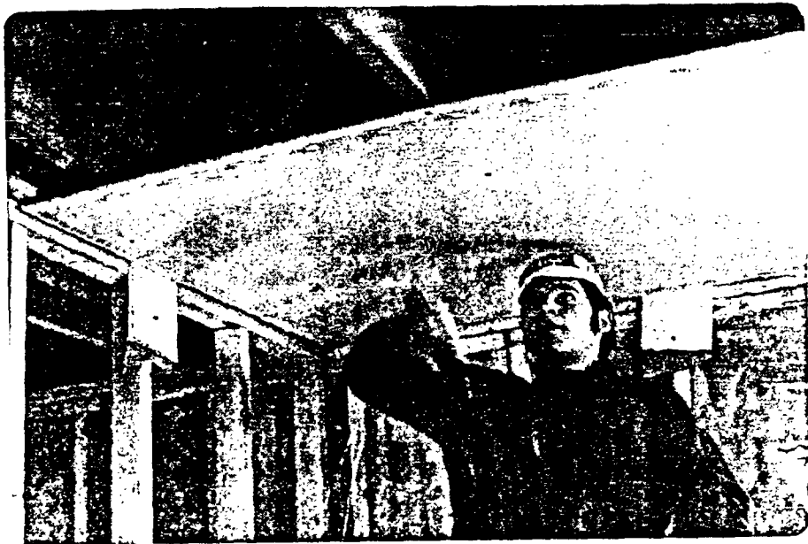
Installation of Panels in Strasburg, Pa. Ranch House
