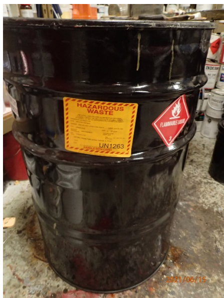
Photo #1 – Open satellite accumulation container in the Chemical Lab.
