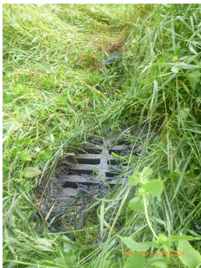
Photo #:17 (P1010218) Description: Northwest storm drain.
