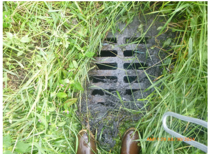
Photo #:16 (P1010177) Description: Northwest storm drain.
