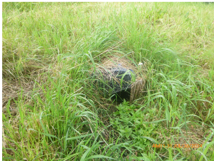
Photo #:20 (P1010223) Description: Manhole where samples are collected.
