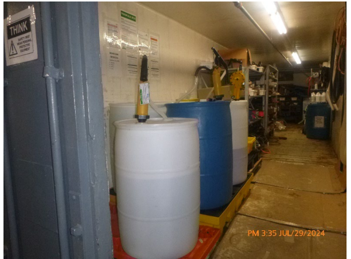
Photo #:08 (P1010196) Description: Chemical storage area
