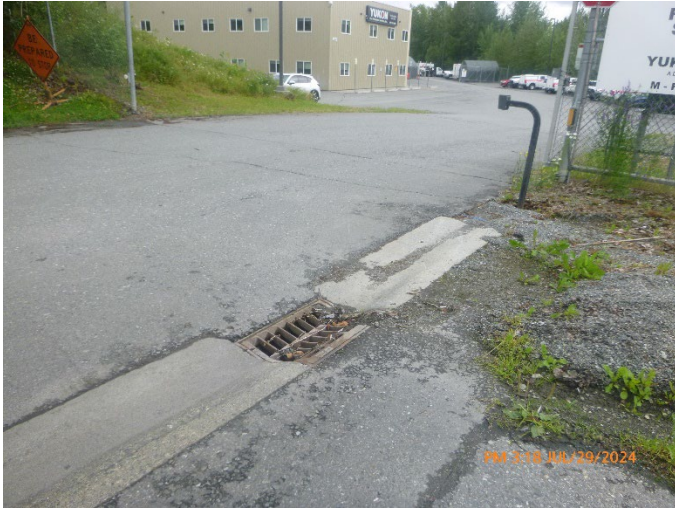
Photo #:21 (P1010180) Description: Storm drain located in the southeast area of the site.
