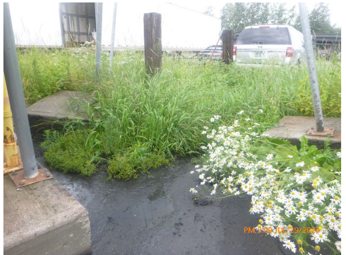
Photo #:12 (P1010170) Description: Northwest storm drain location.
